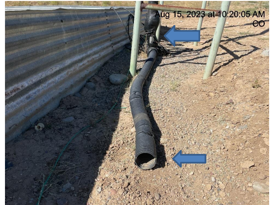
Photo # 5819 Flowline heating insulation open ended
