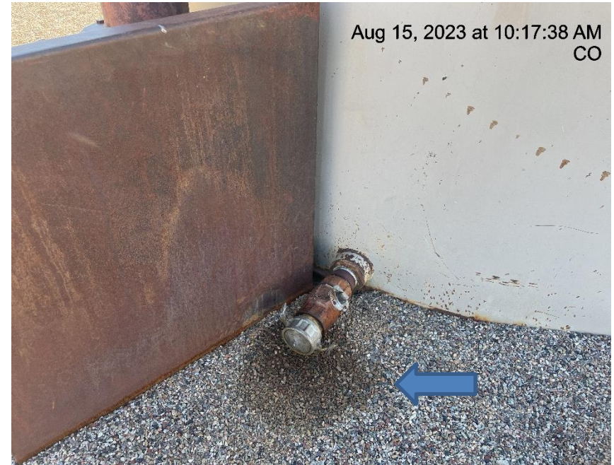
Photo # 5813 Stained gravel in secondary containment
