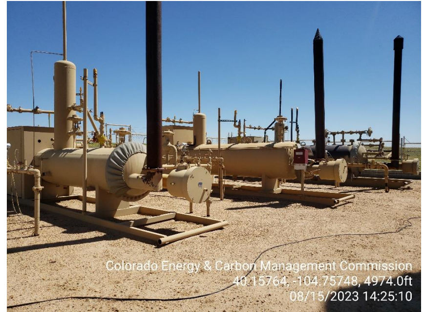
Photo 8 Horizontal Heated Separator.
