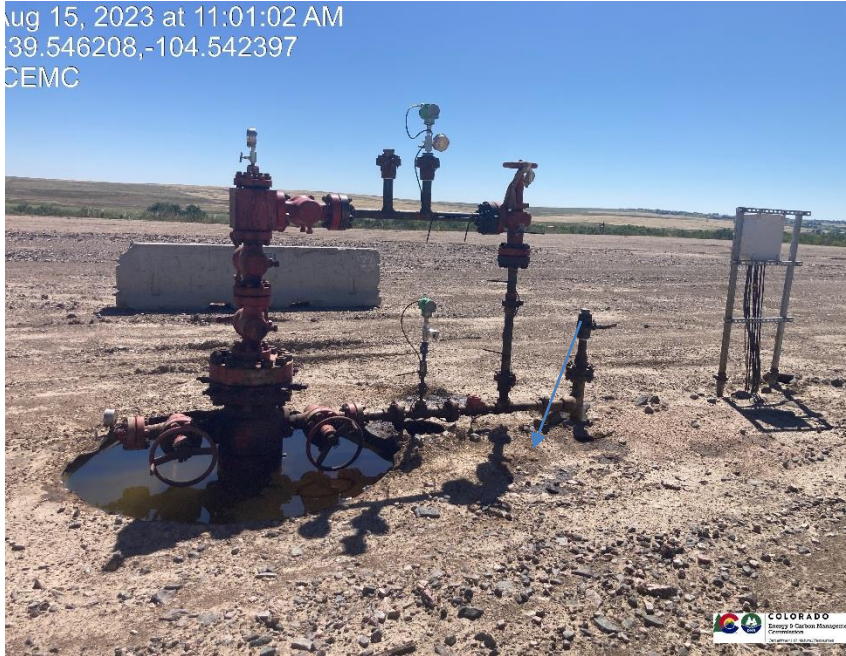
Pic 7 no wellhead sign, contaminated soil needs to be removed from location.
