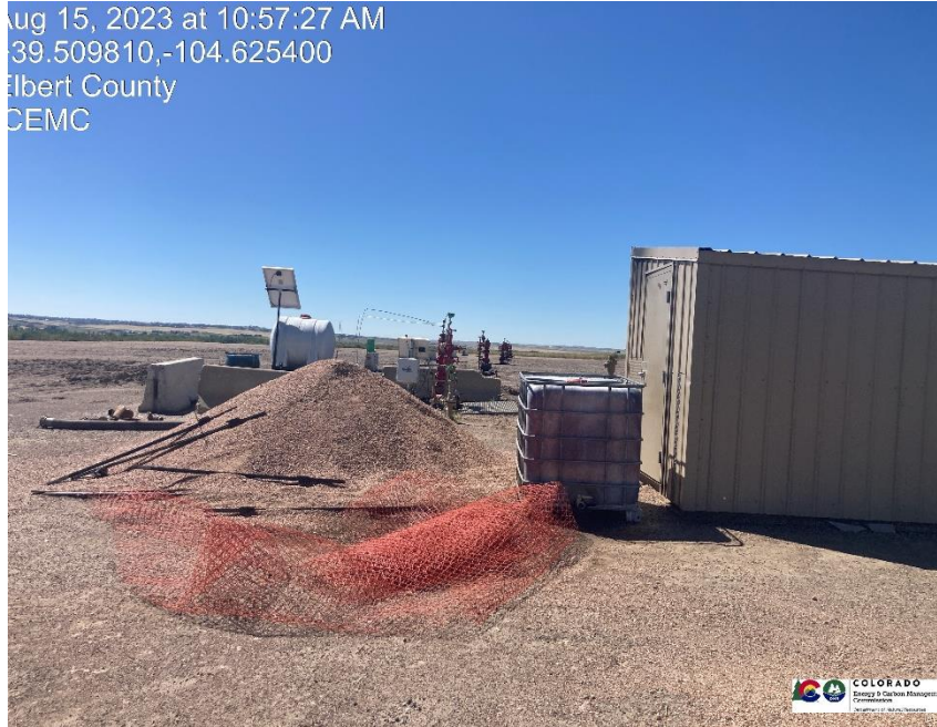
Pic 1 chemical tanks do not have control measures in place to protect from stormwater.
