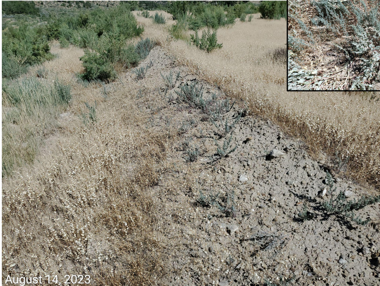
Photo 3: Fill slopes of the Location- Location has not been recontoured, regraded and reclaimed in accordance with 1004 Rules. Halogeton established on Location.
