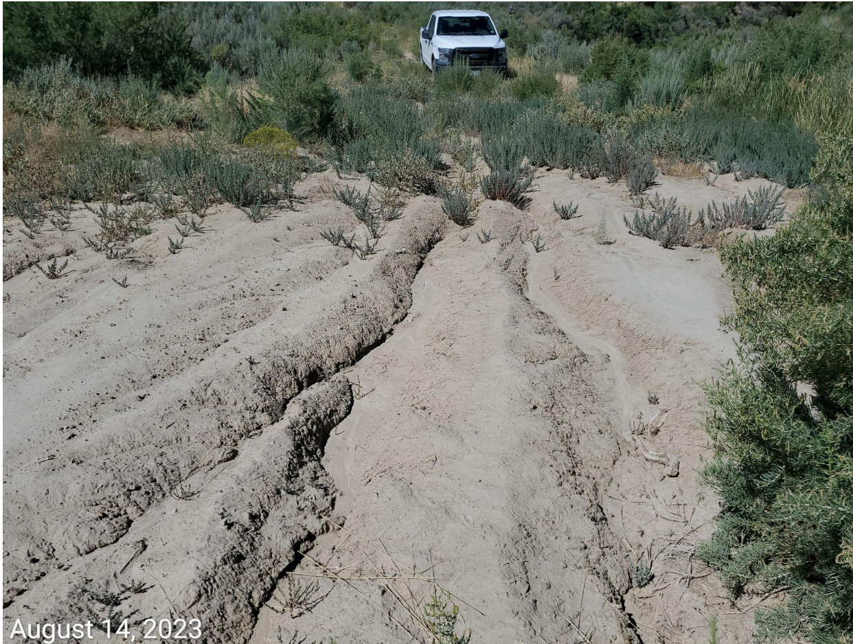
Photo 12: Photo example showing erosion degradation along access road. Stormwater and erosion control measures remain inadequate. Access road has not been decompacted, recontoured, regraded and reclaimed in accordance with 1004 Rules. Photo also shows Halogeton establishment on access road.
