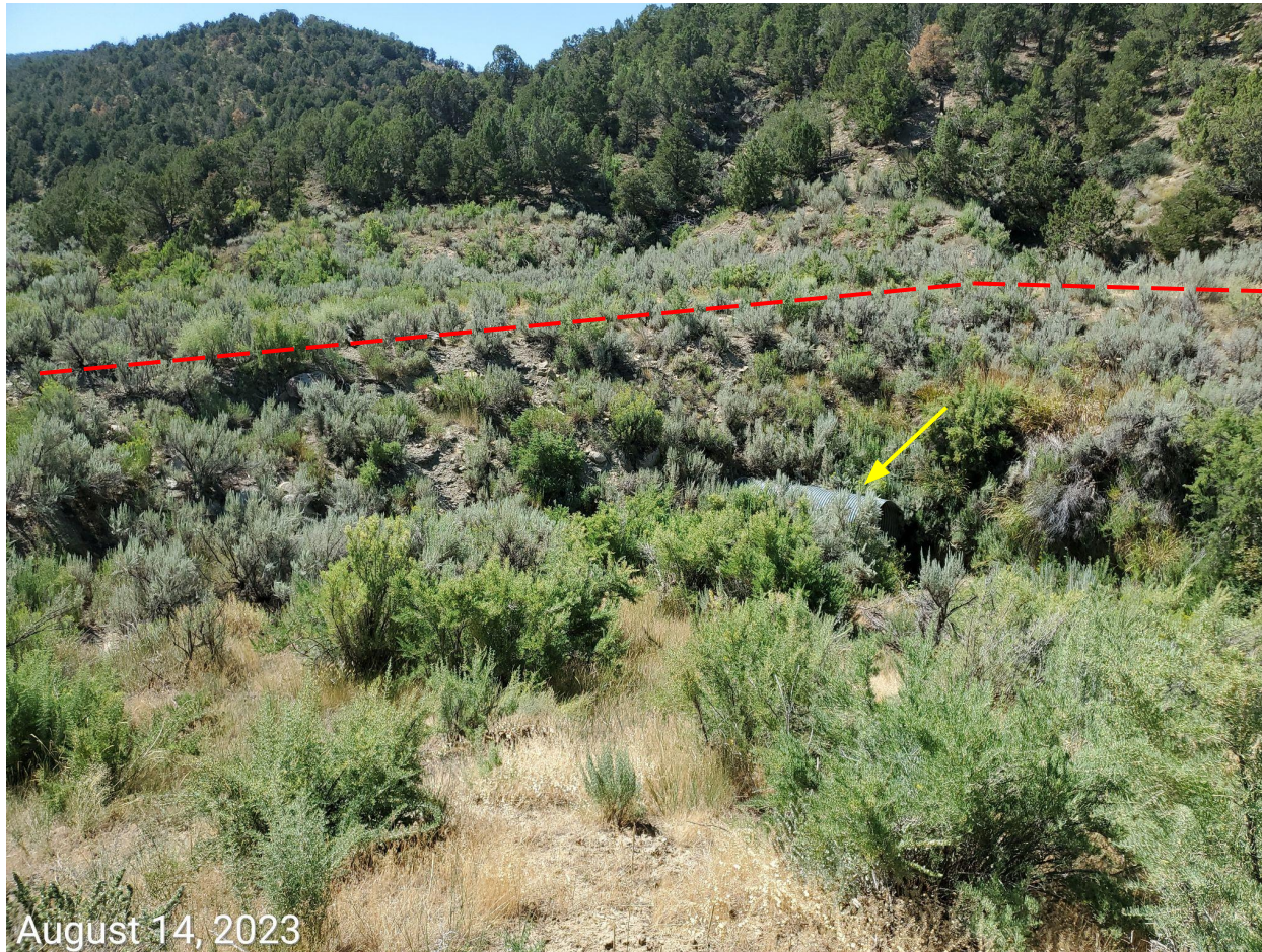
Photo 7: Example of culvert remaining at access road (arrow). Access road (red line) has not been decompacted, recontoured, reggraded and reclaimed in accordance with 1004 Rules; drainage has not been restored
