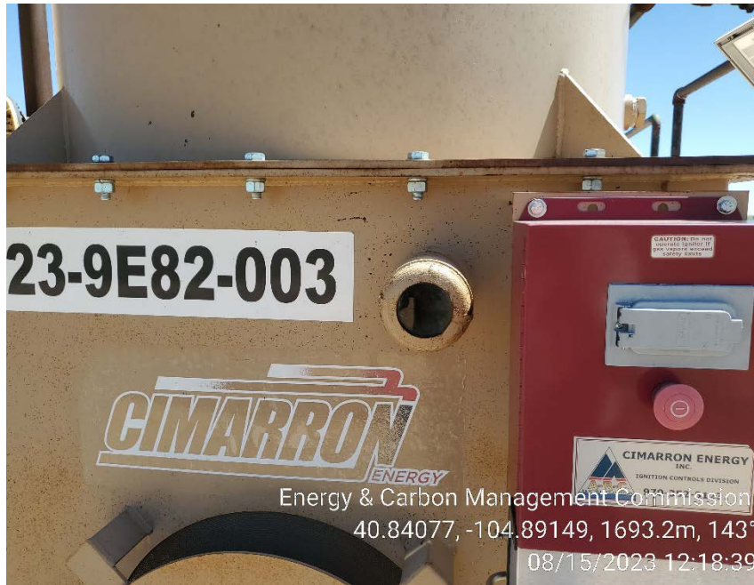
Tank connected inlet open ECD
