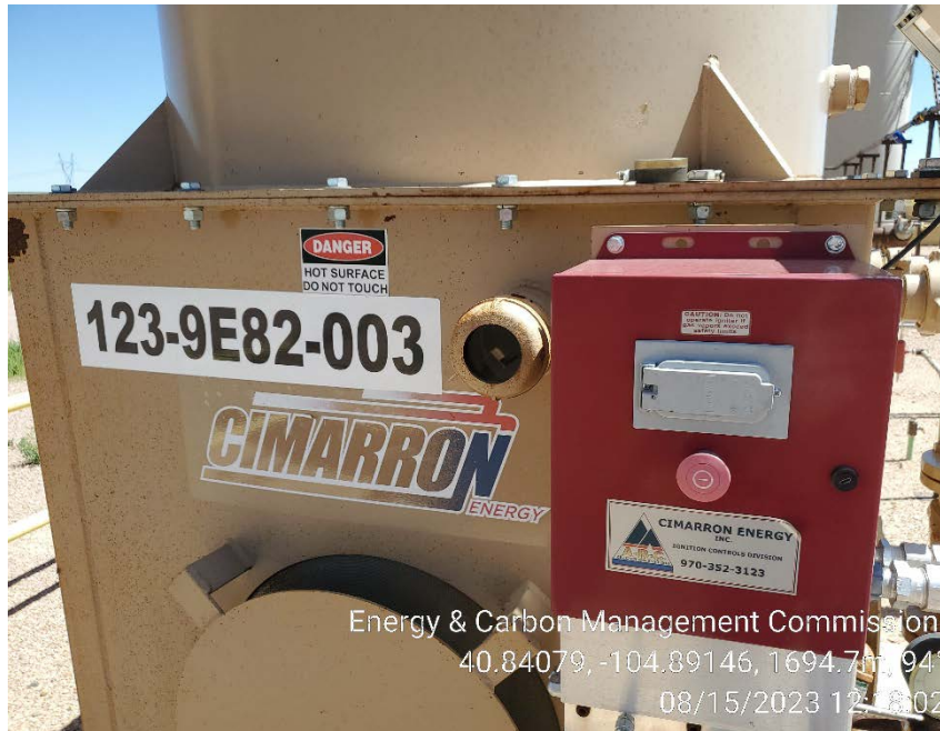
Tank connected inlet shut in ECD
