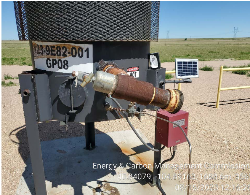
Disconnected ECD with pilot on
