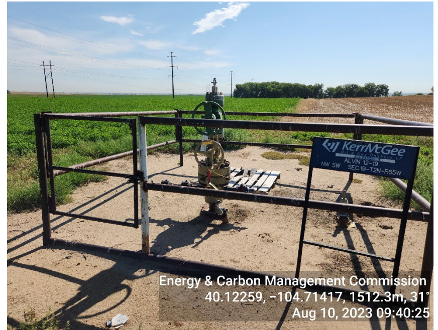
Photo 2: TA Wellhead
