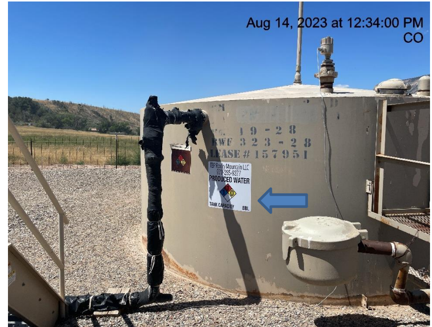
Photo # 5718 Tank label missing required information
