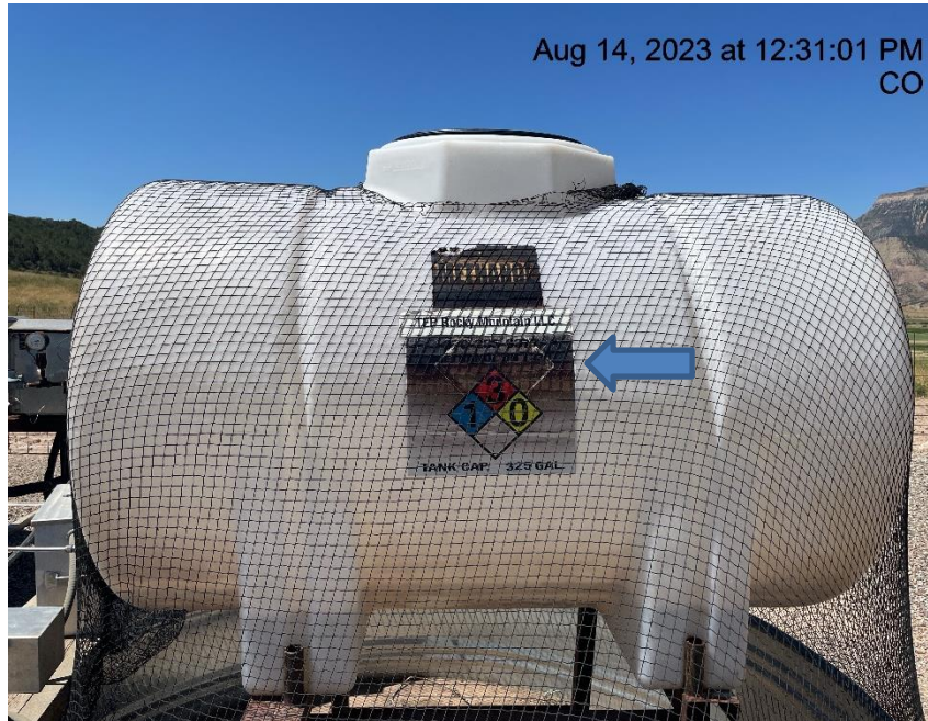
Photo # 5716 Chemical tank label weathered & some info illegible
