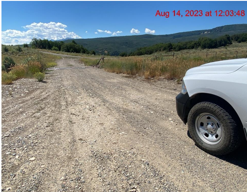
Insufficient Vehicle Tracking BMPs at Location Entrance/Exit – Photo #05814
