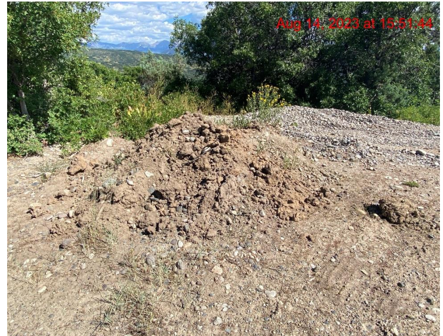
Unprotected Soil Stockpile – Photo #05879
