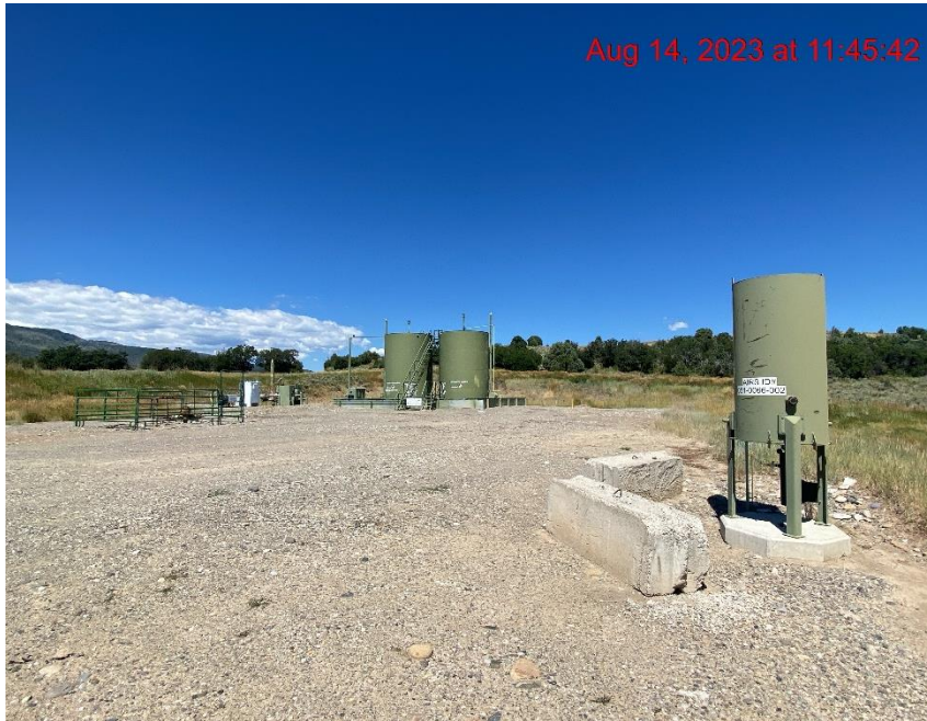
SW Corner of Location – Photo #05802
