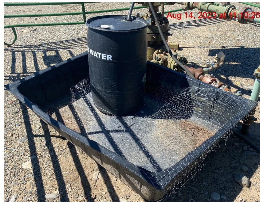
Wildlife Protective Equipment Not Effectively Installed – Photo #05791
