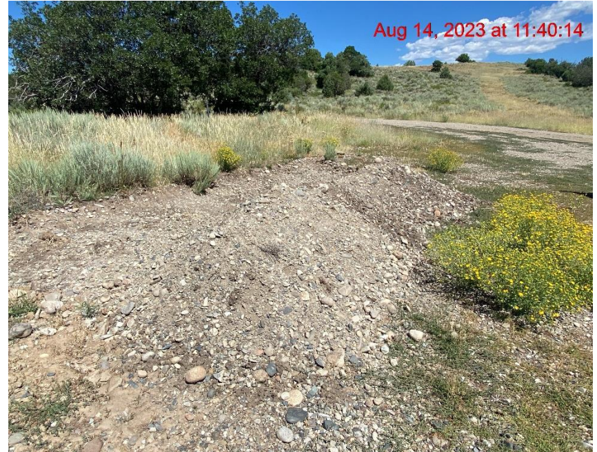
Unprotected Soil Stockpile at Access Road Entrance – Photo #05799
