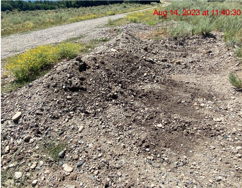
Unprotected Soil Stockpile at Access Road Entrance – Photo #05800
