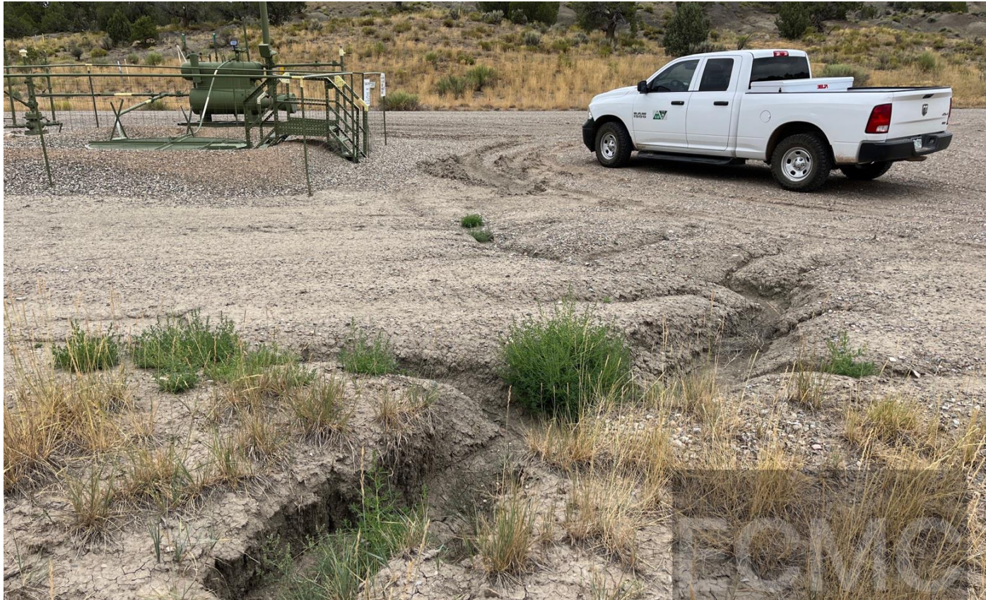
Photo #4. View of gully erosion occurring on location.
