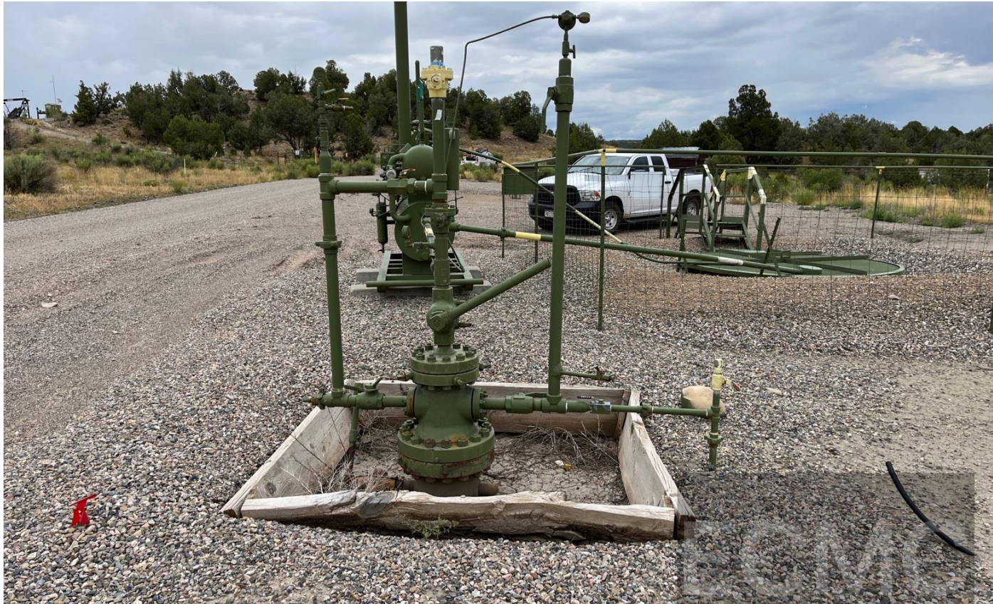
Photo #2. View of the wellhead assembly.
