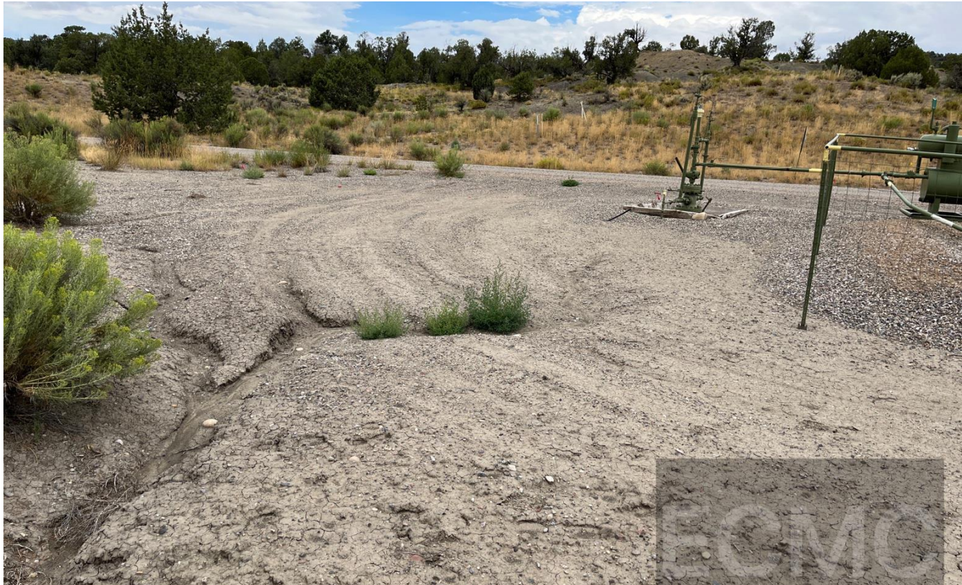
Photo #5. View of gully erosion occurring on location.
