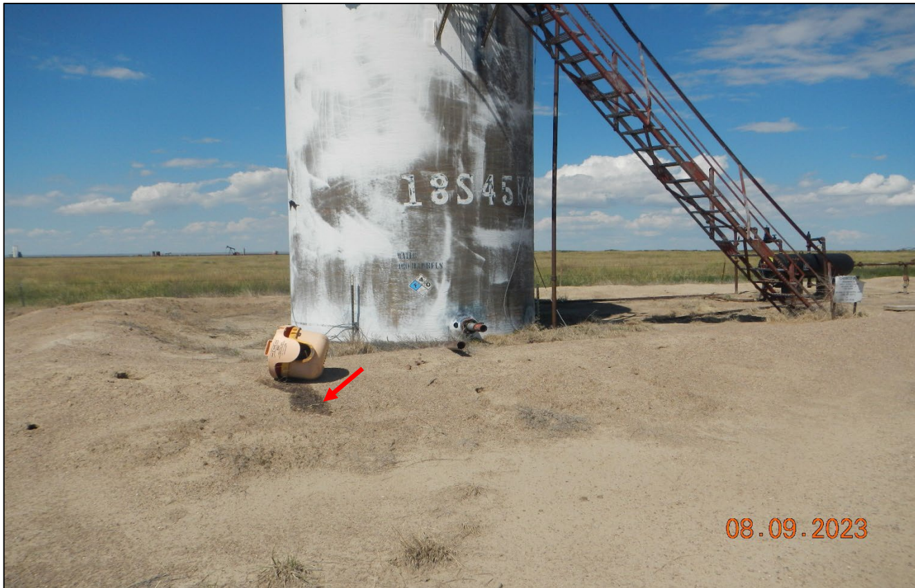
Photo 2. Facing northeast toward the tank battery. There is oil stained soil at red arrow that needs to be cleaned up. Berm does not appear to be adequate for containment.
