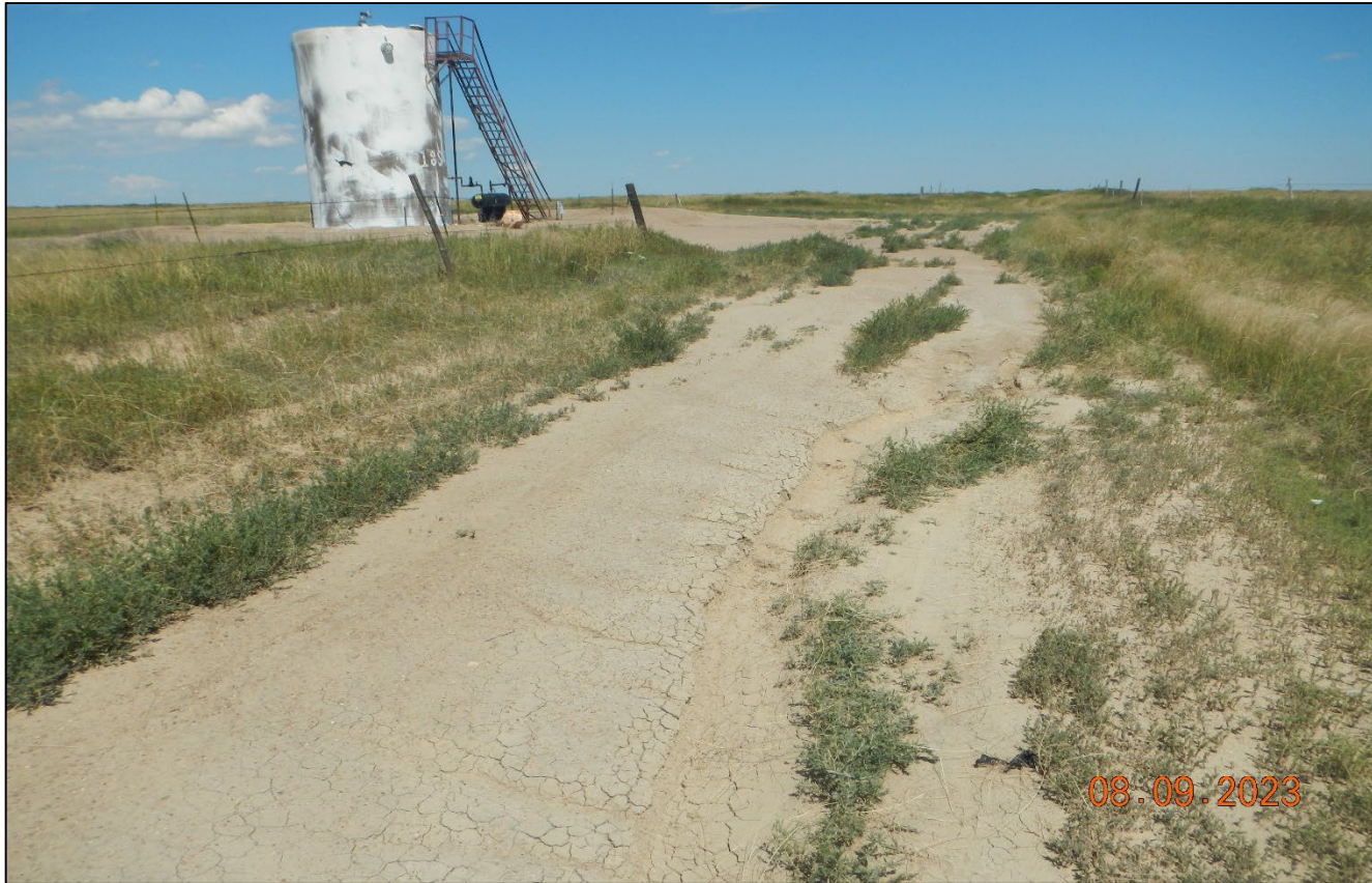
Photo 1. Facing east near the tank battery. There is erosion along the access road in this area that needs to be repaired.
