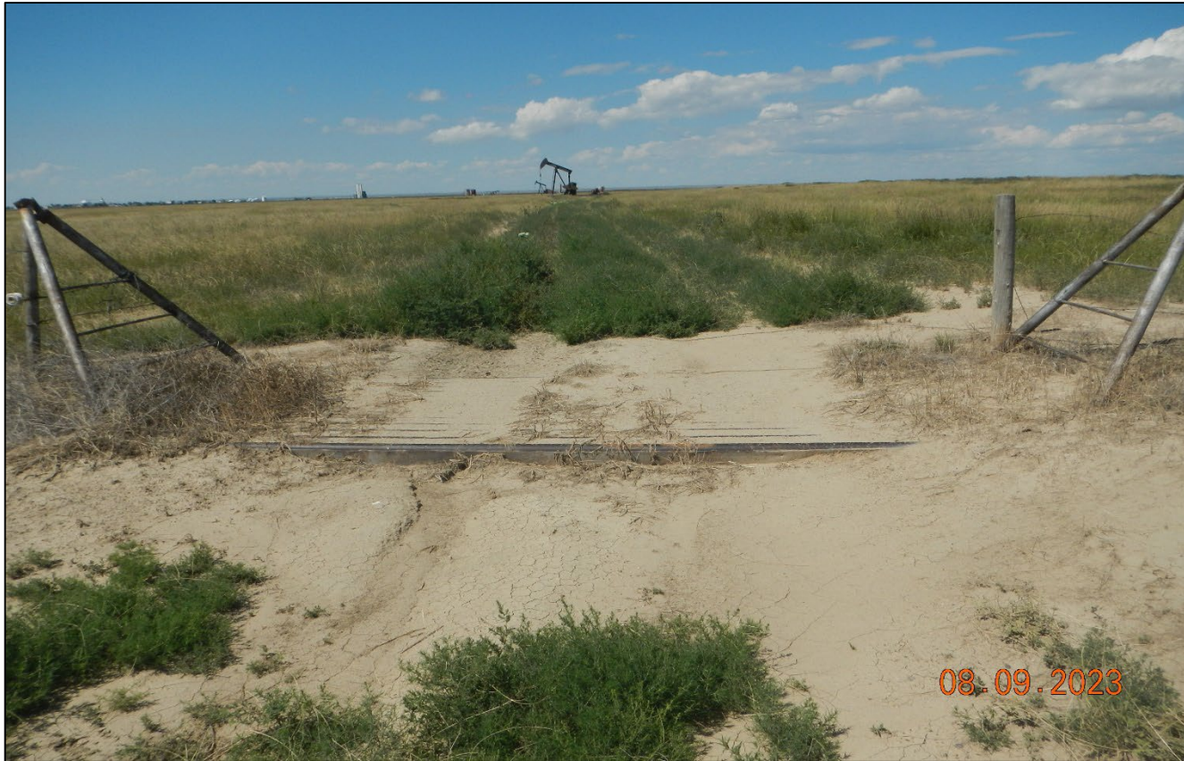
Photo 3. Facing north along the access road. The cattle guard is filled in with sediment and needs maintenance.
