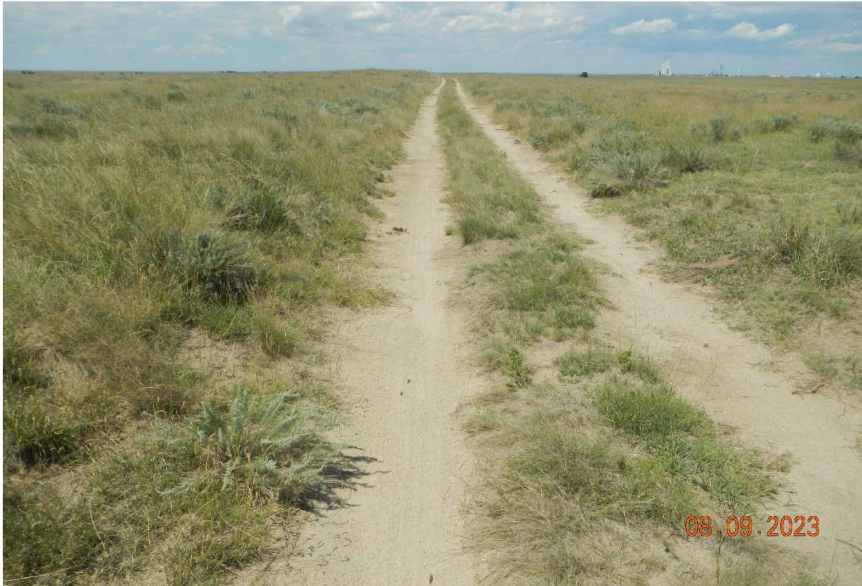
Photo 1. Facing north along the access road. This portion of the road has not been recontoured and reclaimed. Previous corrective action not completed.
