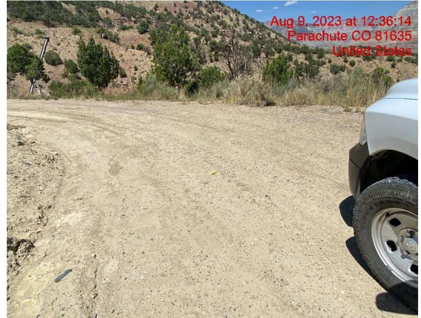
Insufficient Vehicle Tracking BMPs at Location Entrance/Exit – Photo #05766
