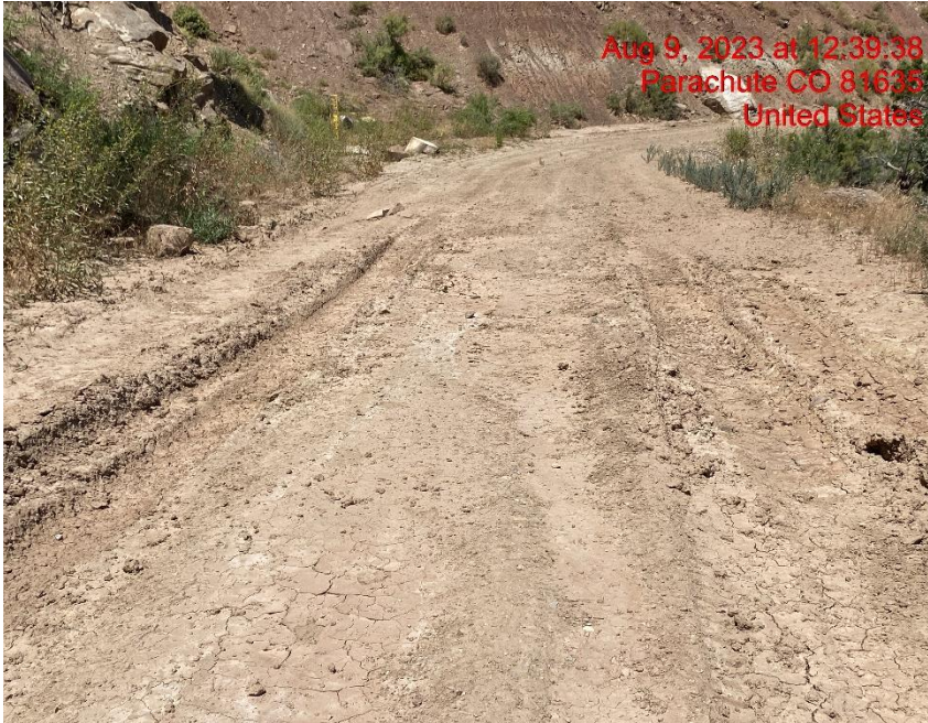
Lease Road Lacks Stabilization – Photo #05770
