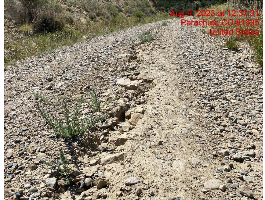
Rill Erosion Cutting Through Lease Road – Photo #05769
