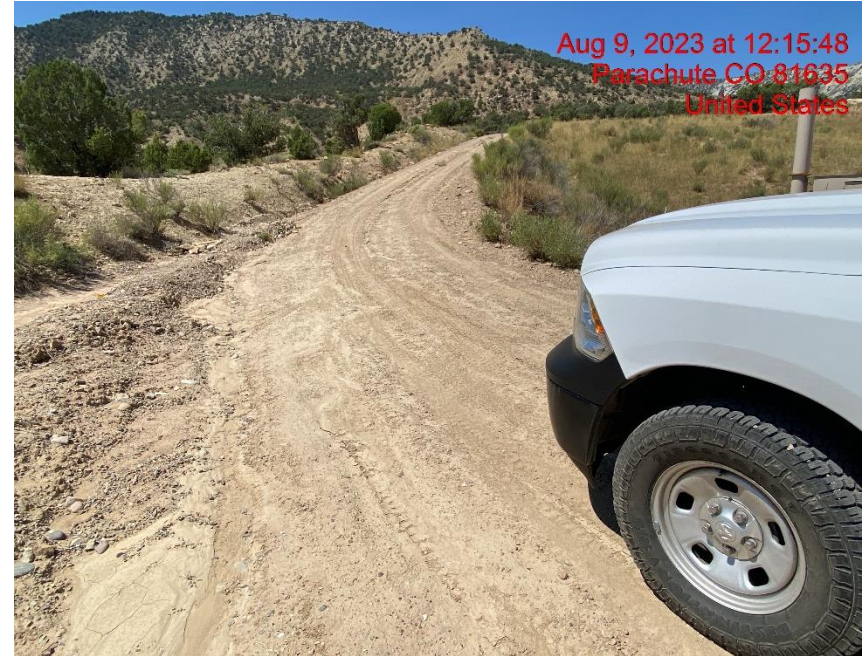
Insufficient Vehicle Tracking BMPs at Location Entrance/Exit – Photo #05754
