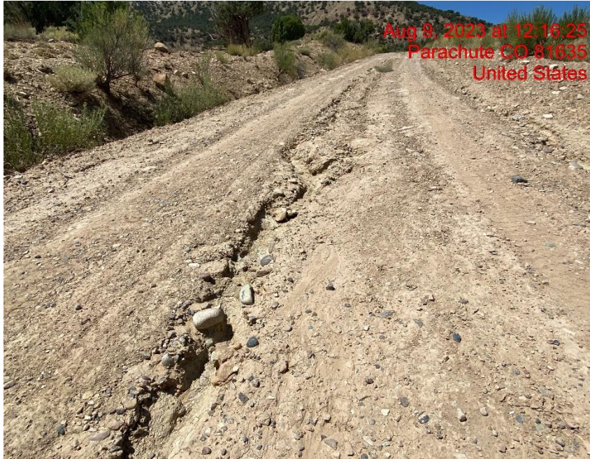
Rill Erosion Cutting Through Lease Road – Photo #05756
