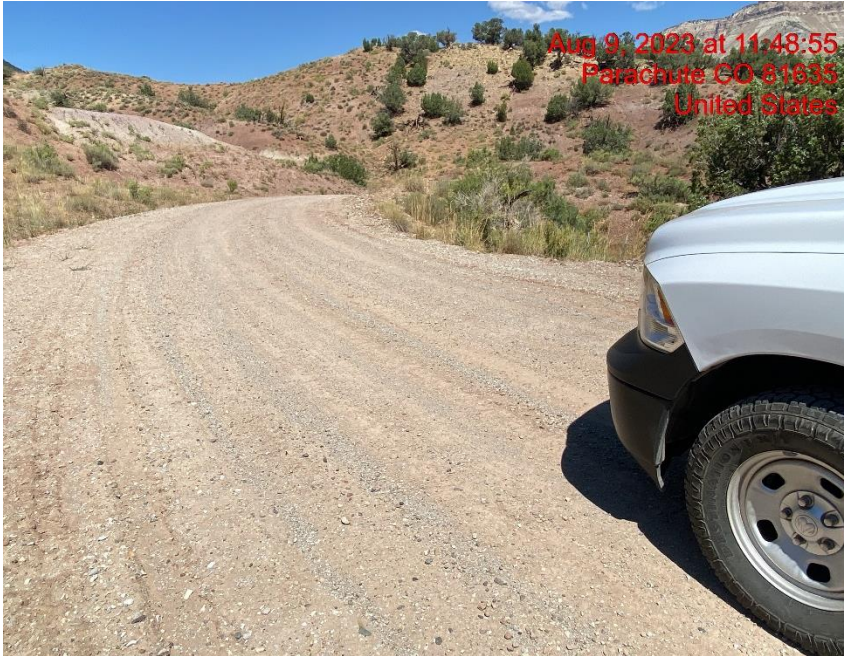
Insufficient Vehicle Tracking BMPs at Location Entrance/Exit – Photo #05745
