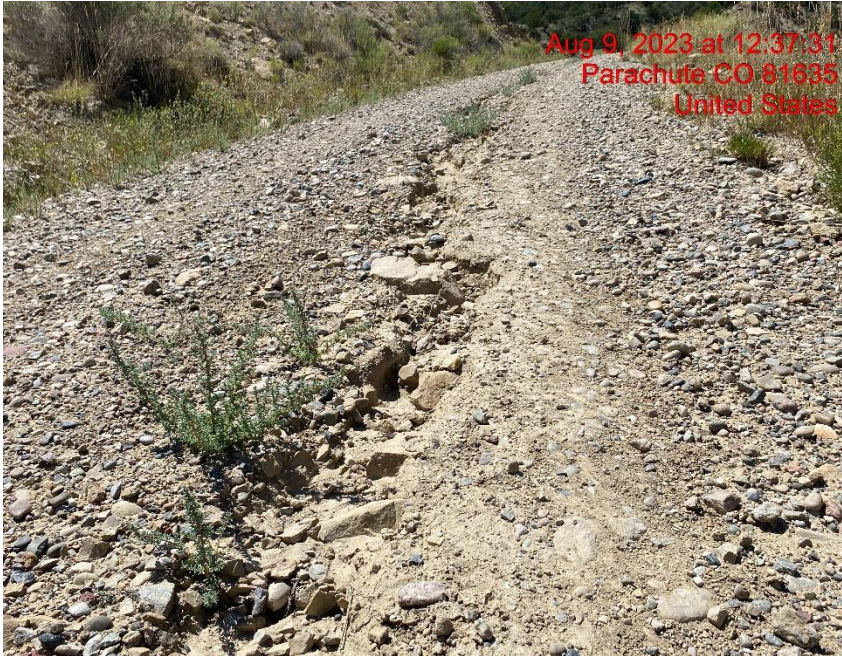
Rill Erosion Cutting Through Lease Road – Photo #05769
