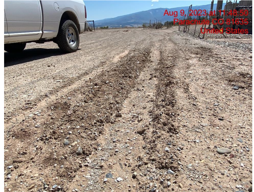
Location Lacks Stabilization – Photo #05744
