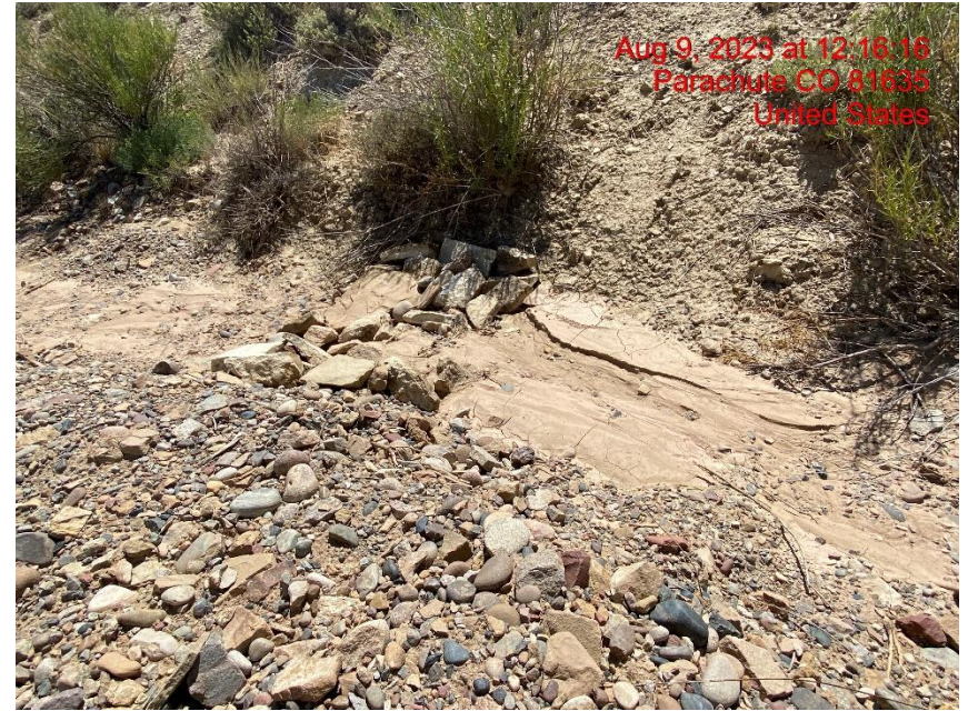
Check Dam Needs Maintenance – Photo #05755
