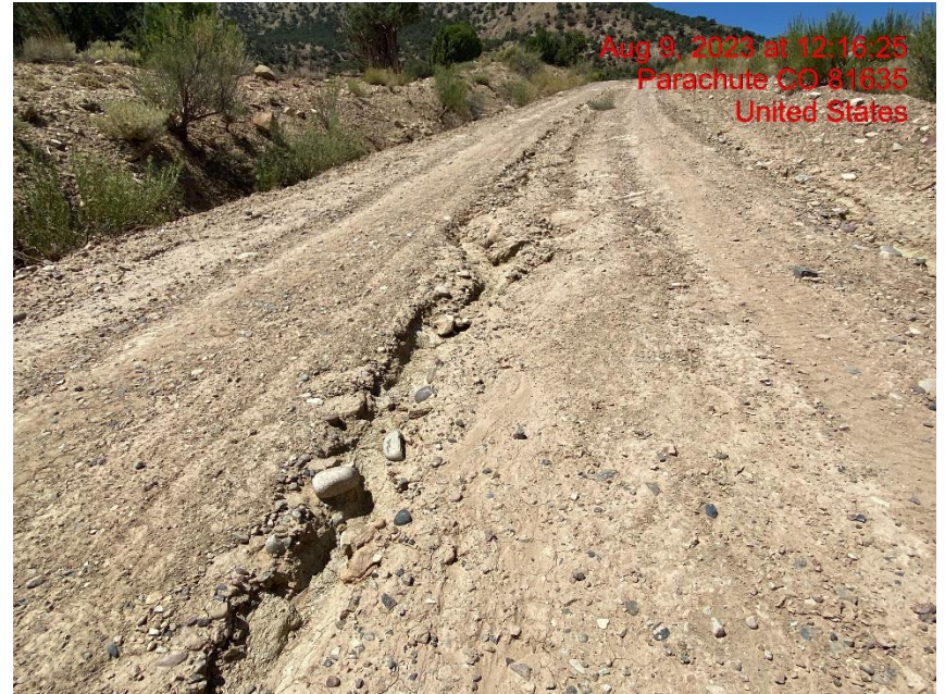
Rill Erosion Cutting Through Lease Road – Photo #05756
