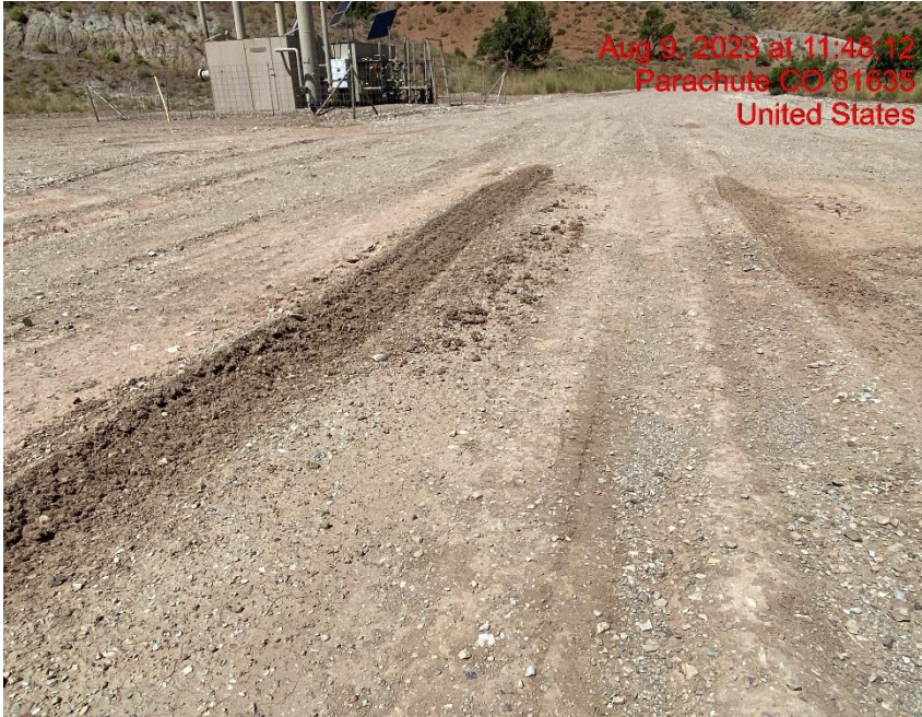
Location Lacks Stabilization – Photo #05743
