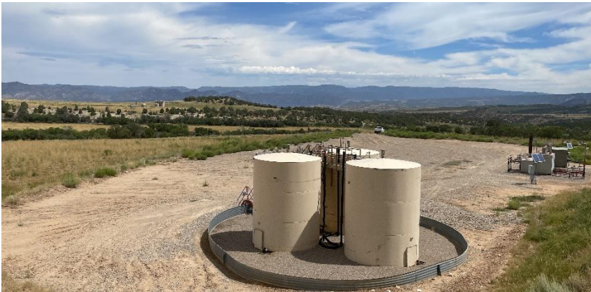
South West corner of location.
