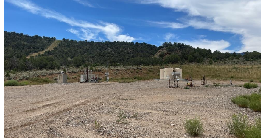
North East corner of location.
