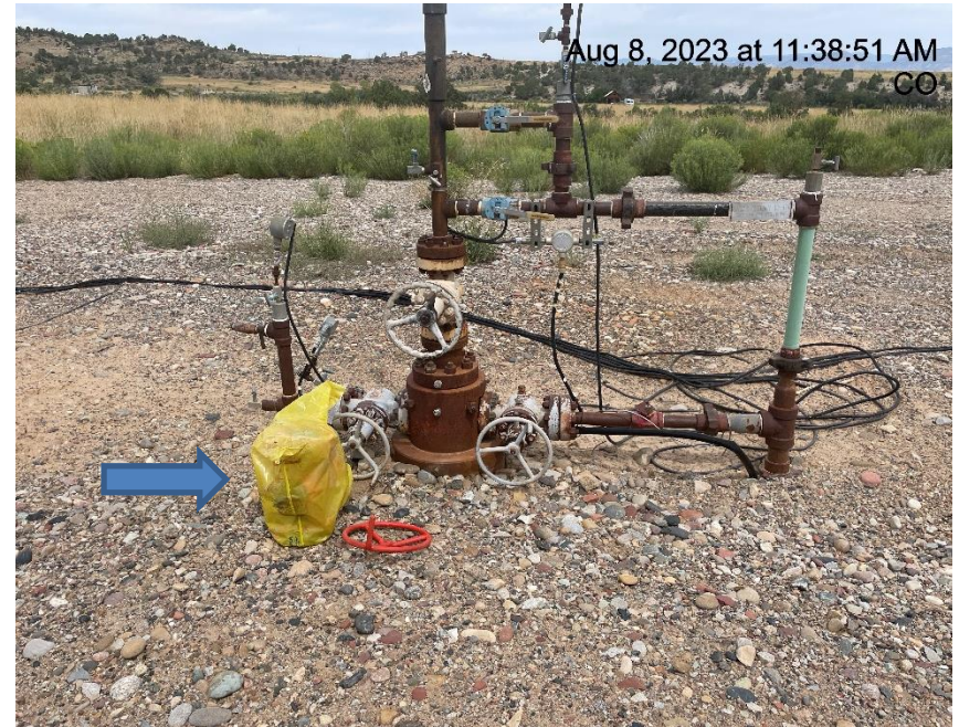
Photo # 5329 Unused equipment/supplies
