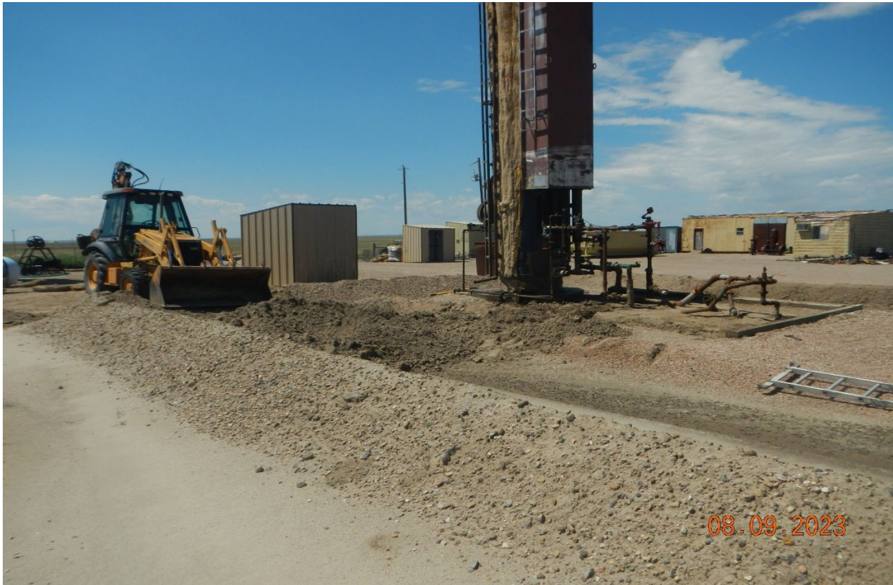
Photo 5. Facing northwest toward the vertical separator. The shed has been removed and there is excavation and work being performed at the separator.
