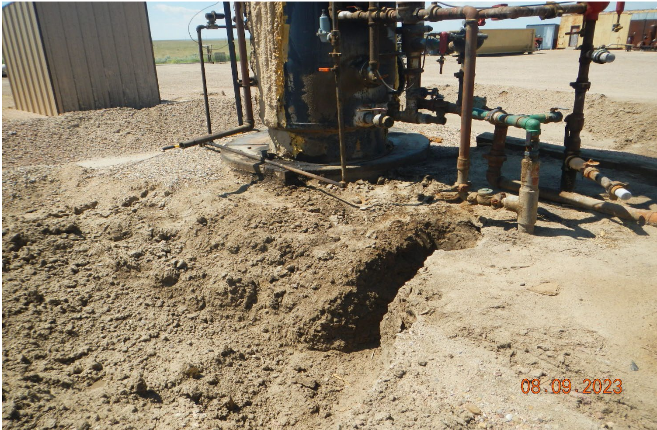
Photo 6. View of excavation and exposed piping at separator. There is oil stained soil observed in this area that will need to be cleaned up.
