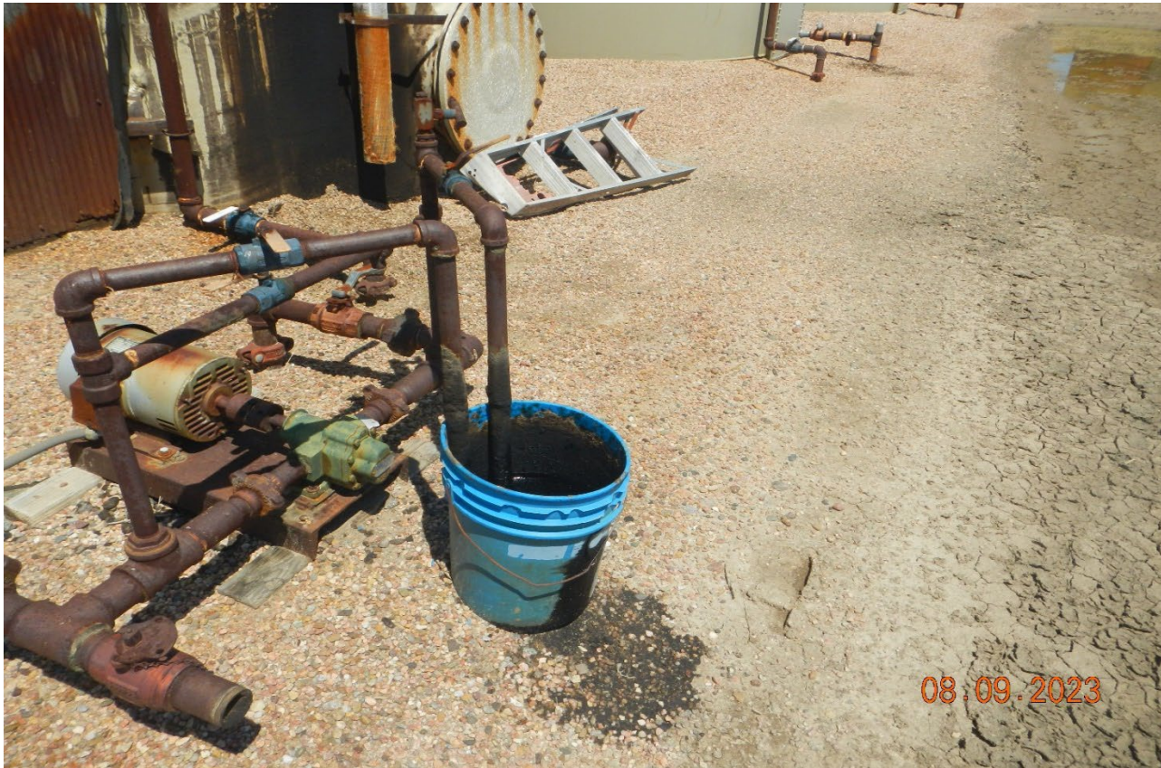
Photo 8. This bucket at the backside of the tank battery is full of oil which has spilled onto the ground. This needs to be cleaned up and covered to prevent entry.
