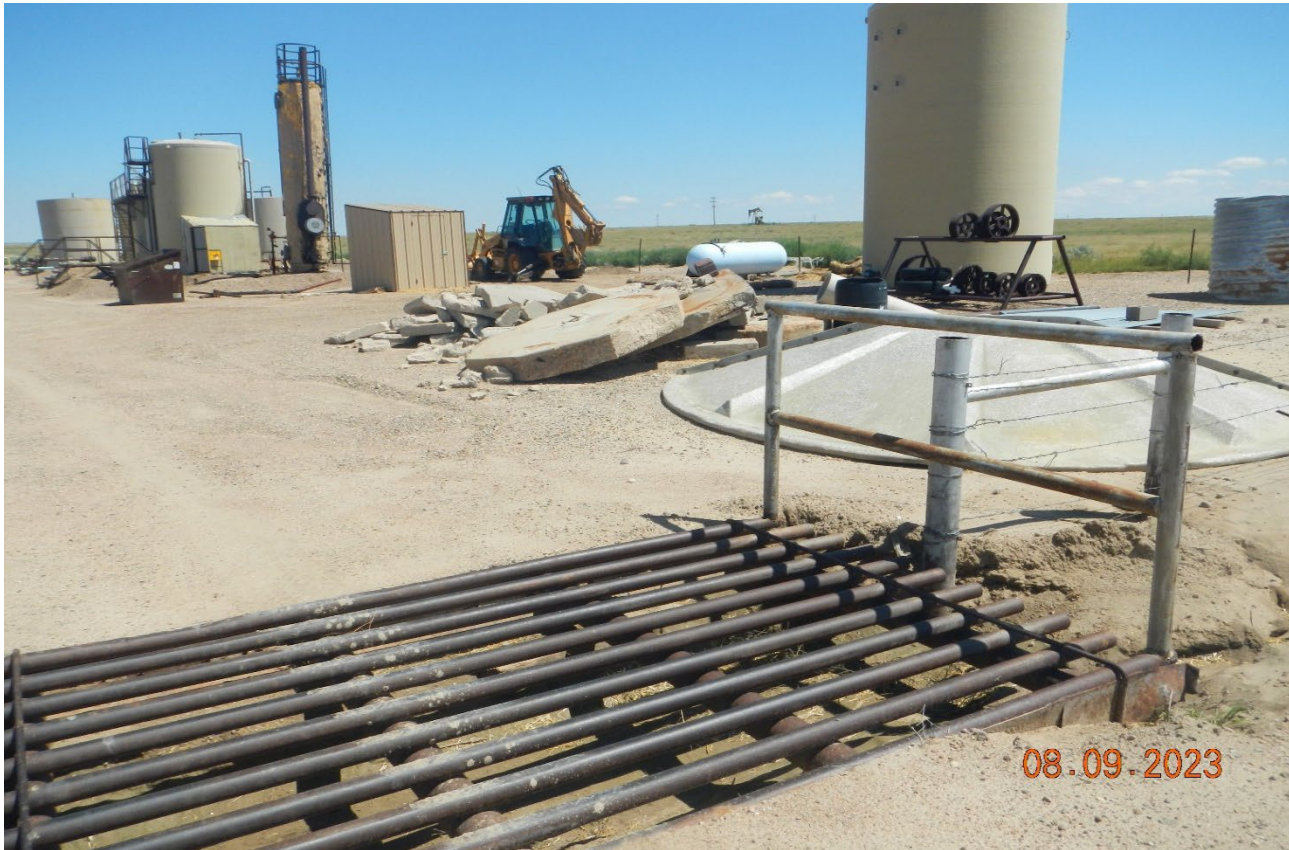
Photo 11. Facing southeast toward the PYLES offsite tank battery and storage yard. There is concrete debris and a broken bottom of a tank among other debris and equipment that must be removed per Rule 606 & 1003.a.
