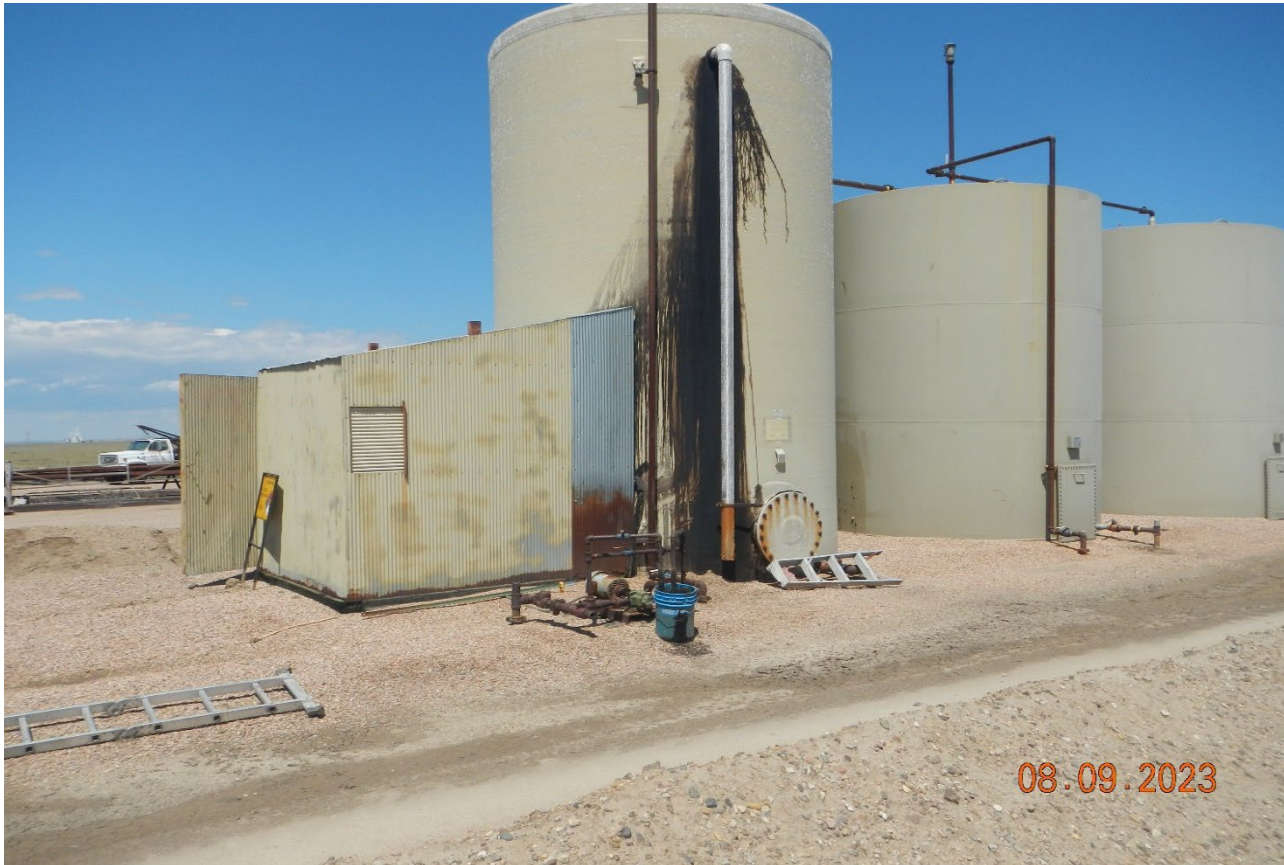
Photo 7. Facing at the back side of the tank battery. There was a spill from the tank which needs to be cleaned up. The blue bucket needs to be emptied and disposed of any oil. Previous corrective action was not completed.
