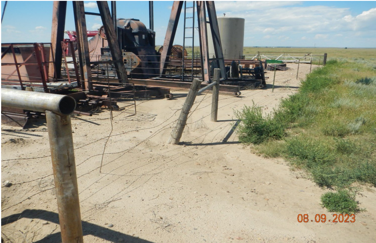
Photo 20. East side of the location at the cattleguard. The fence in this area has a large gap and may not prevent livestock entry. This area needs to be repaired.
