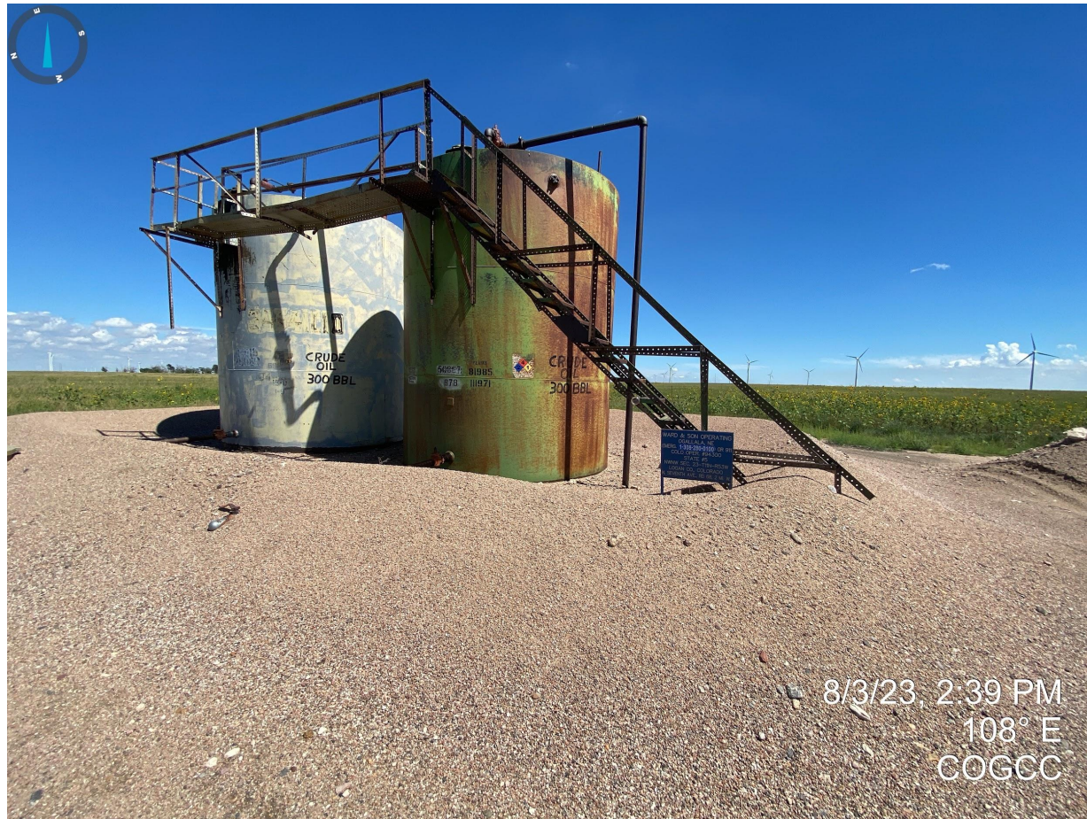
Photo 10. Secondary containment around the tank battery does not appear adequate to contain 150% of the volume of the largest tank.
