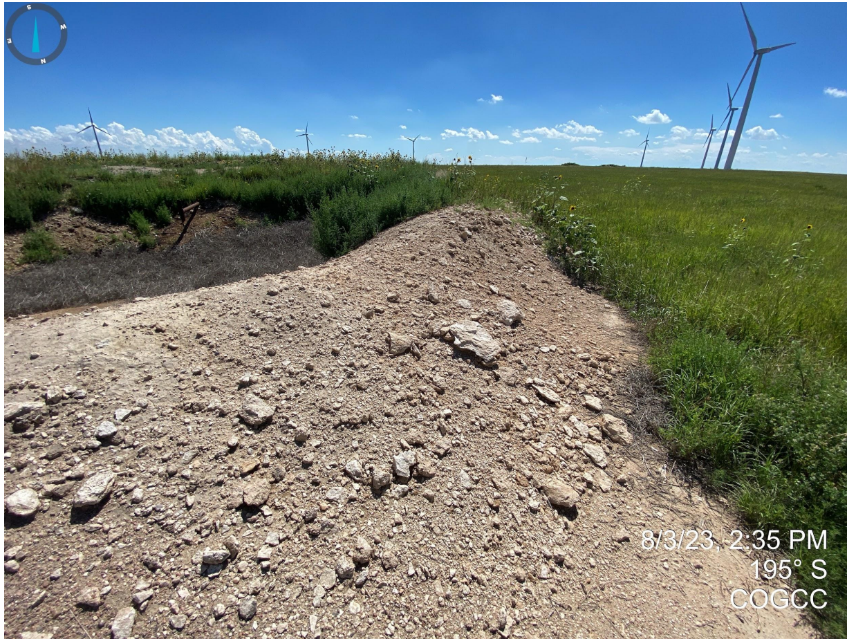
Photo 1. Plt walls/berms appear to be comprised of unconsolidated material and are not properly stabilized.
