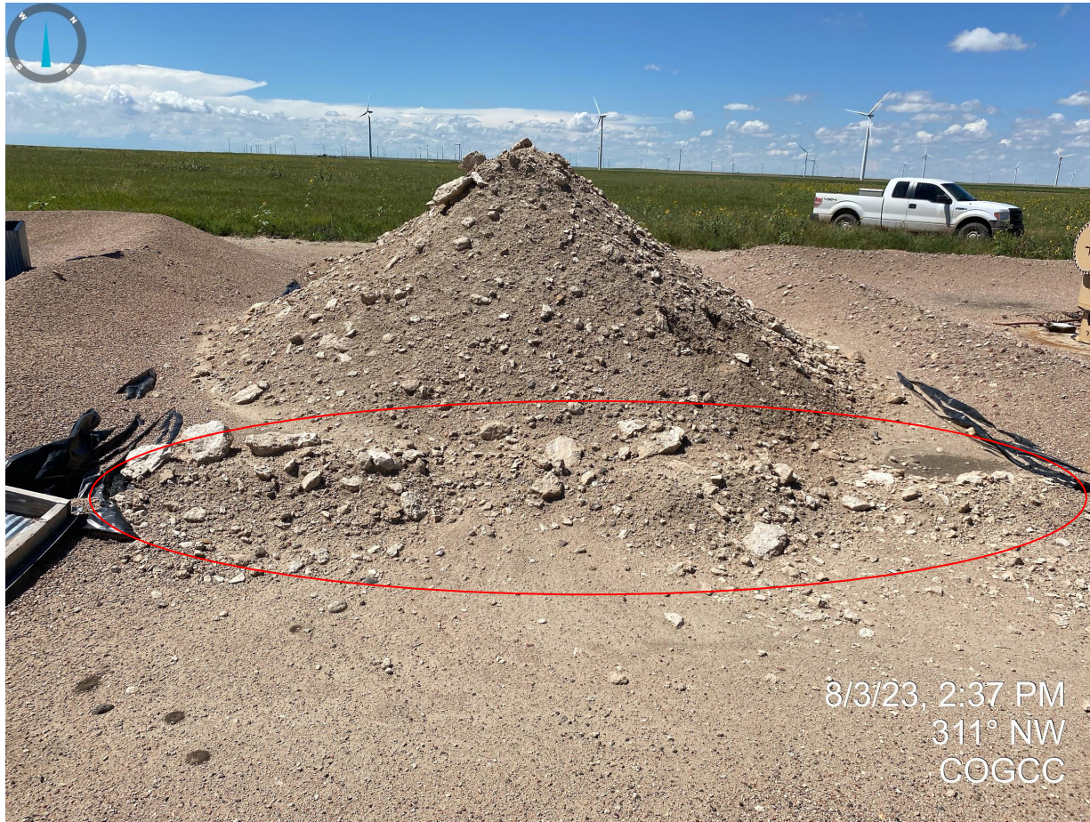
Photo 7. Apparent impacted material does not have adequate secondary containment.
