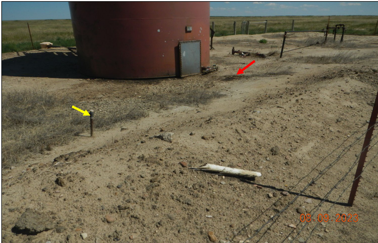
Photo 2. There is oil stained soils near the tank at the red arrow. There is an unused pipe riser at the yellow arrow and various plastic debris.
