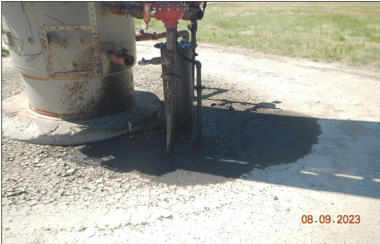
Photo 4. There is oil saturated soils at the base of the separator approximately 4ft. X4ft. Oil soils need to be cleaned up.
