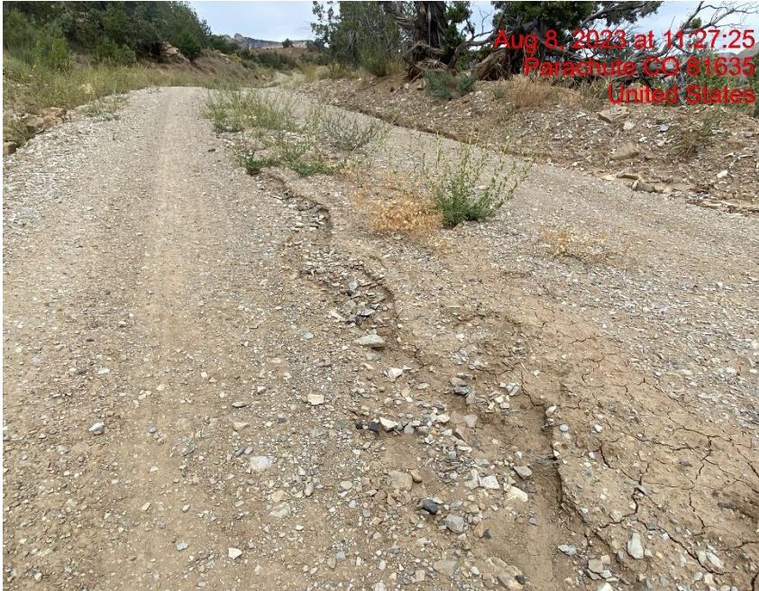
Rill Erosion Cutting Through Lease Road – Photo #05693
