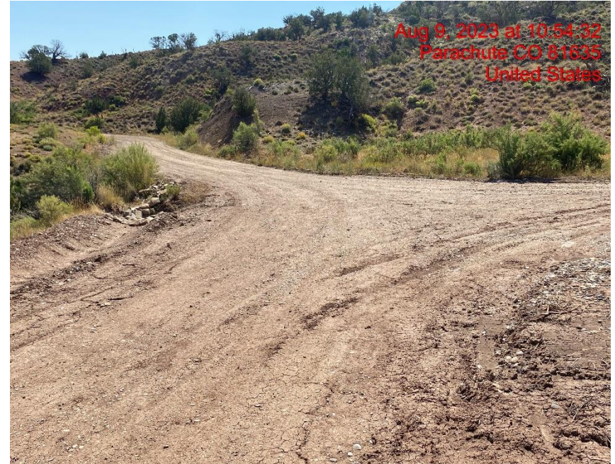
Insufficient Vehicle Tracking BMPs at Location Entrance/Exit – Photo #05718
