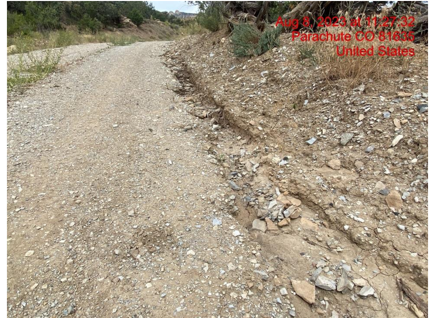
Rill Erosion Cutting Through Lease Road – Photo #05694
