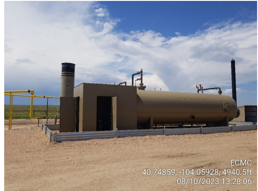
Photo 6 – ECD and Separator
