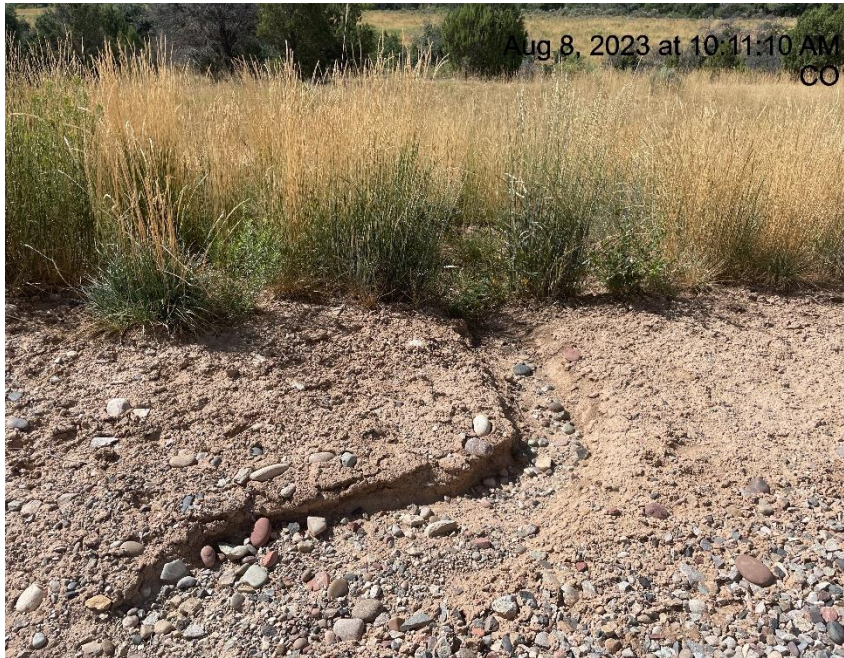
Photo # 5198 Erosion & transport of sediment off location into vegetation (near production separators)
