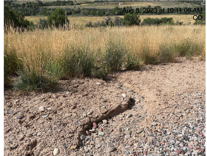
Photo # 5197 Erosion & transport of sediment off location into vegetation (near production separators)
