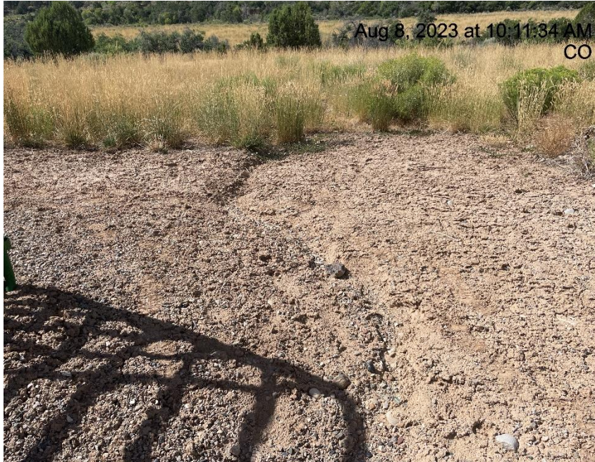
Photo # 5196 Erosion & transport of sediment off location into vegetation (near production separators)
