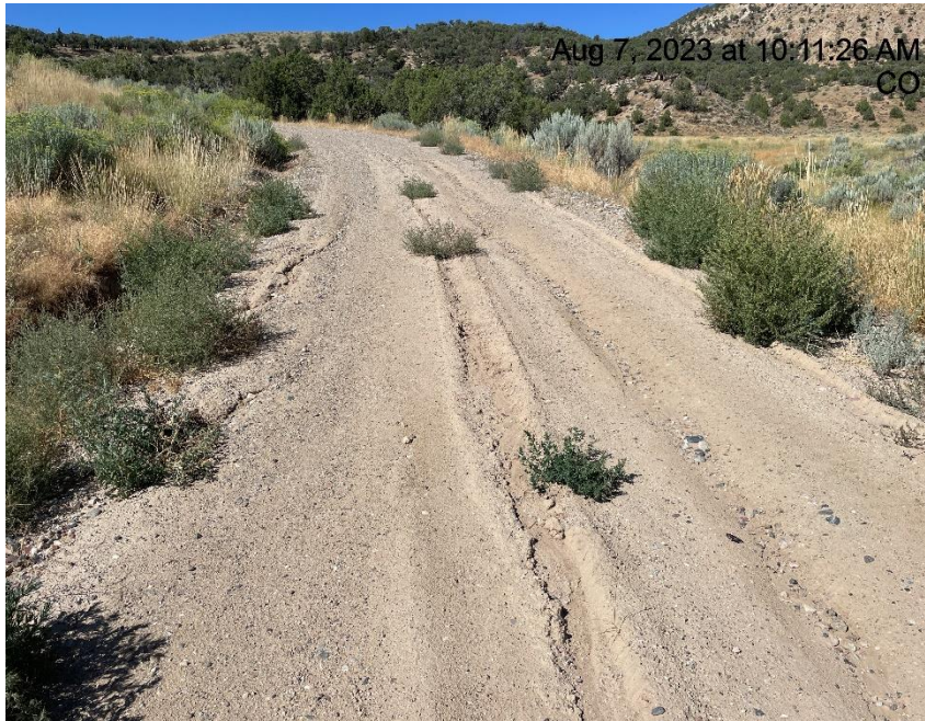
Photo # 4893 Erosion & transport of sediment on lease road
