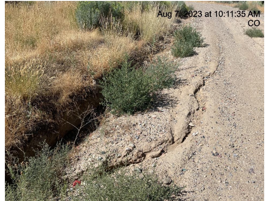
Photo # 4894 Erosion & transport of sediment on lease road
