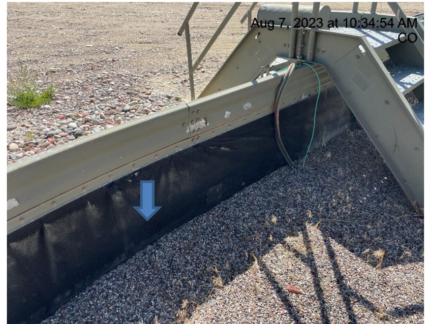
Photo # 4952 Secondary containment liner needs maintenance
