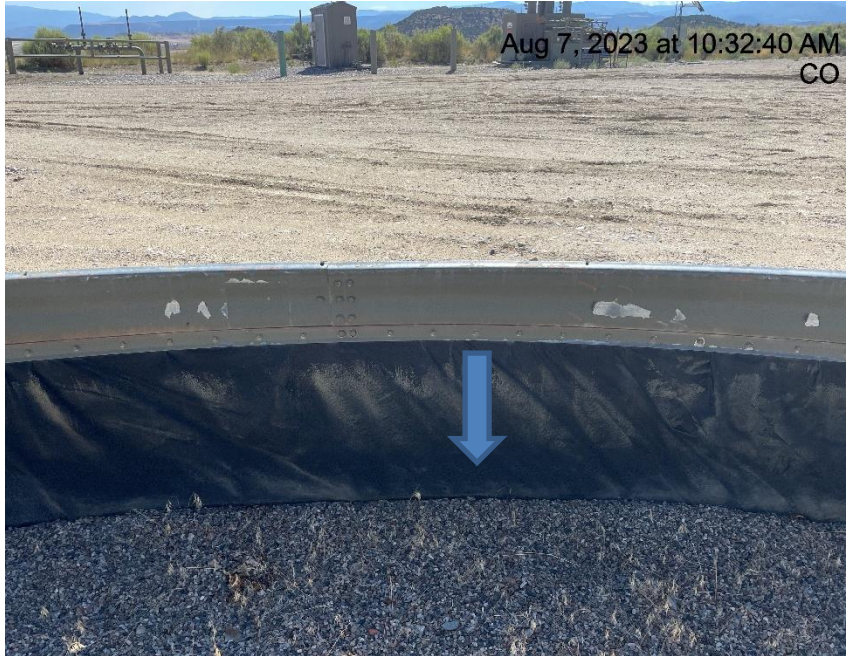
Photo # 4934 Secondary containment liner needs maintenance
