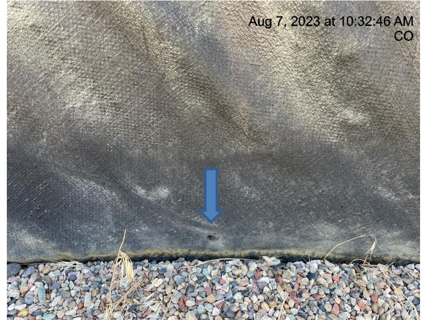
Photo # 4988 Secondary containment liner needs maintenance
