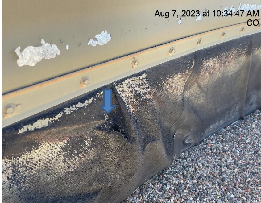
Photo # 4951 Secondary containment liner needs maintenance
