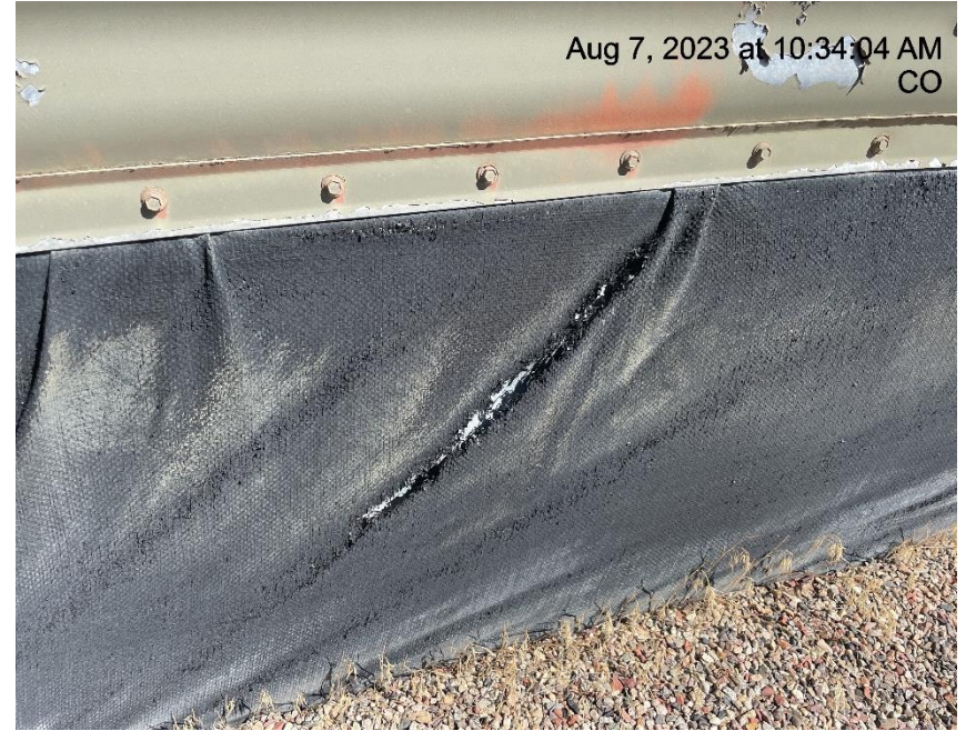
Photo # 4944 Secondary containment liner needs maintenance
