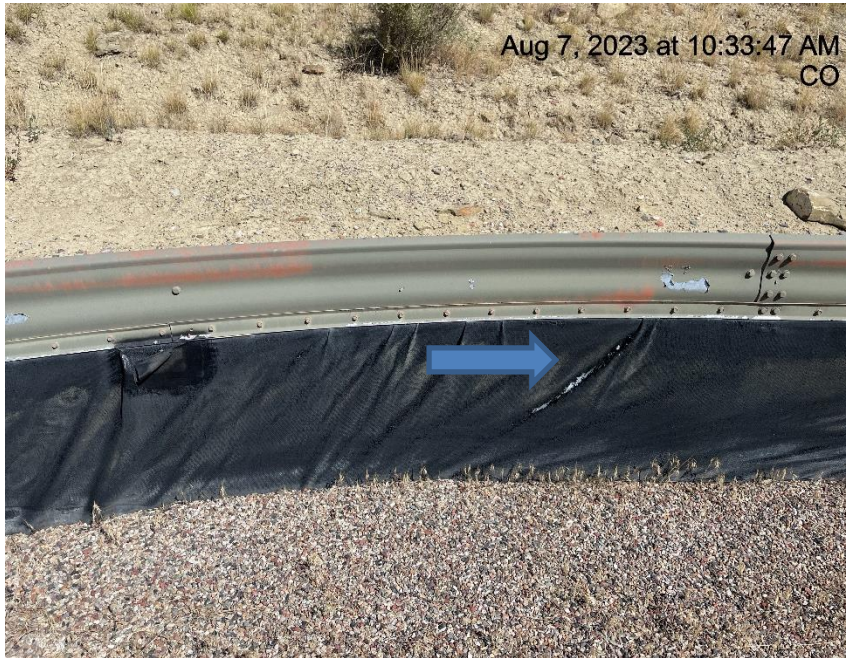
Photo # 4941 Secondary containment liner needs maintenance
