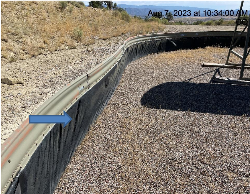
Photo # 4943 Secondary containment liner needs maintenance
