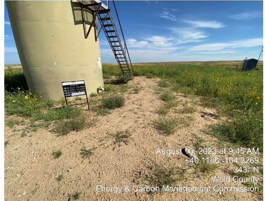
Overgrown Vegetation & Weathered Berms
