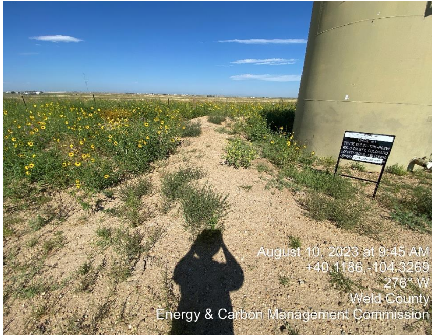
Overgrown Vegetation & Weathered Berms
