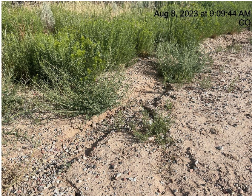
Photo # 5120 Erosion & transport of sediment off location into vegetation (west side of pad)
