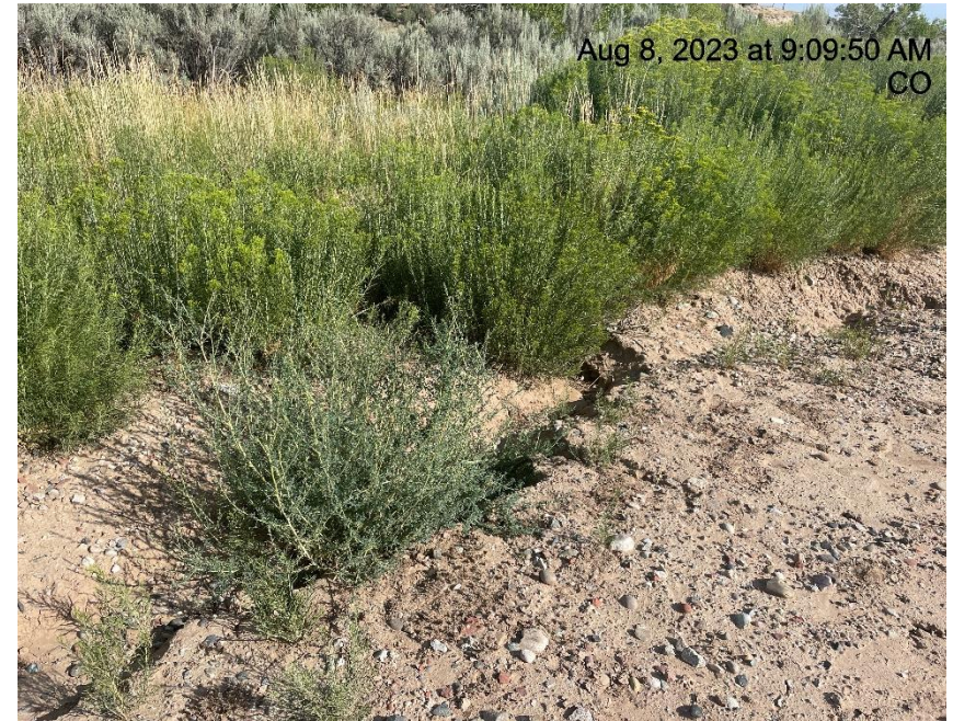
Photo # 5121 Erosion & transport of sediment off location into vegetation (west side of pad)
