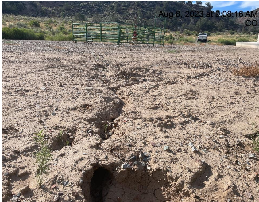
Photo # 5117 Tunnel erosion (Near edge of pad near separator unit & Summit meter house)
