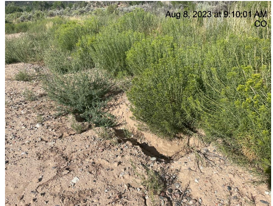
Photo # 5123 Erosion & transport of sediment off location into vegetation (west side of pad)
