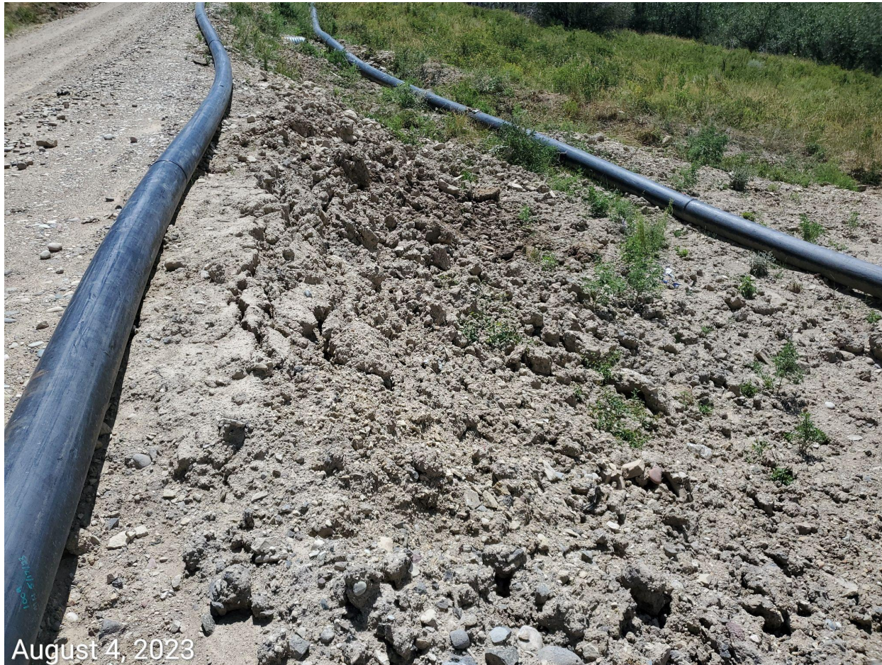
Photo 8: Stormwater and erosion control measures to minimize erosion and degradation missing or insufficient at slopes adjacent to Location entrance; slopes lack stabilization.
