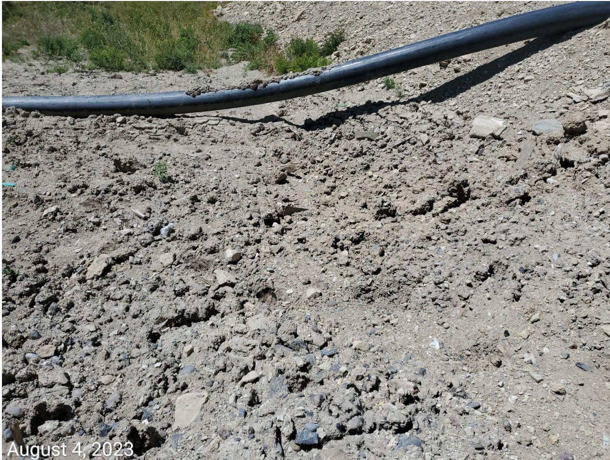
Photo 9: Stormwater and erosion control measures to minimize erosion and degradation missing or insufficient at slopes adjacent to Location entrance; slopes lack stabilization.
