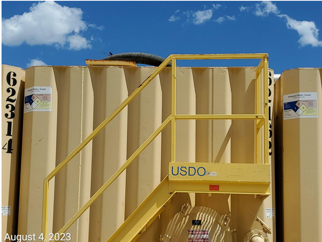
Photo 4: Photo example showing containers missing labeling information per 605 Rules.
