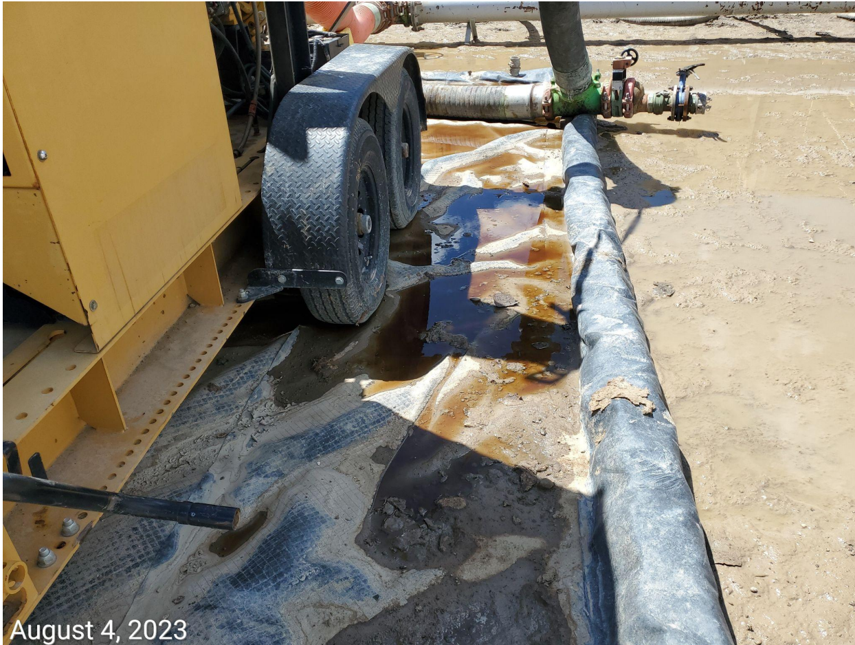
Photo 7: Fluids in containment require removal and proper disposal.
