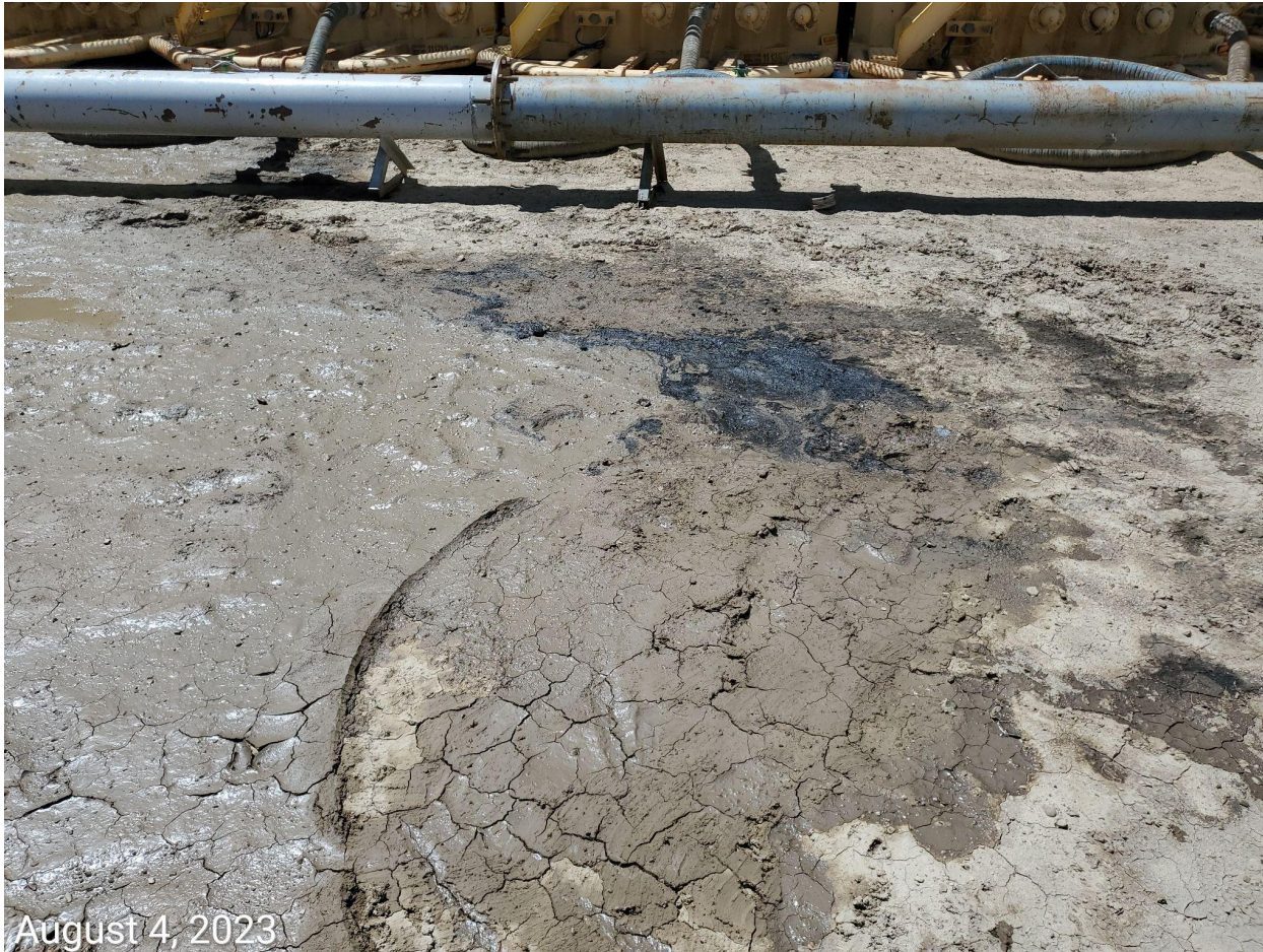
Photo 6: Recent winds have blown over a portable light unit, resulting in POLS spilling onto the working pad surface, and impacting stormwater.
