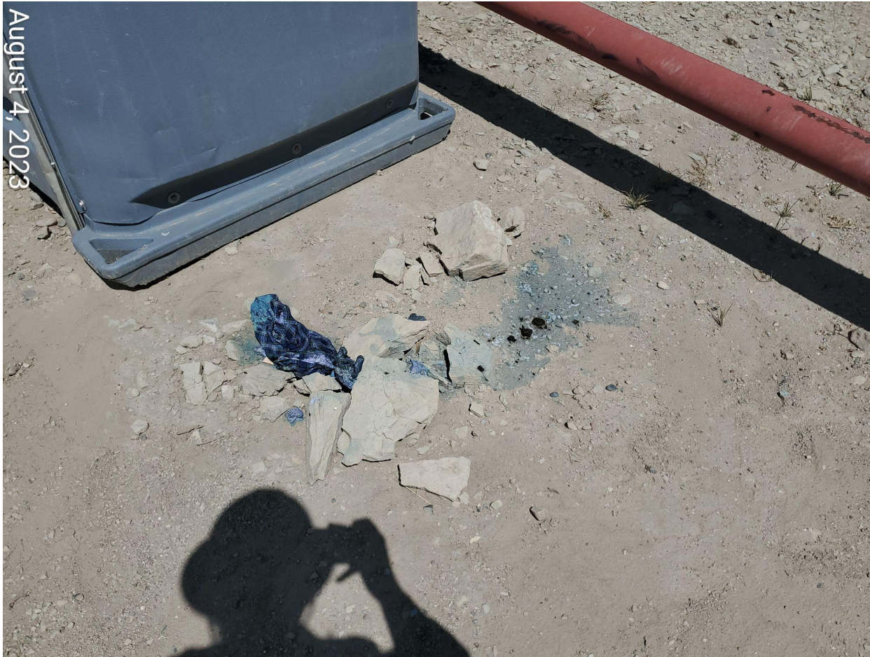
Photo 2: Continued from photo 1. Photo shows that BMPs to ensure that waste remains contained within the sanitary facilities is inadequate; chemicals and fecal material observed spilled onto the working pad surface next to porta-john.
