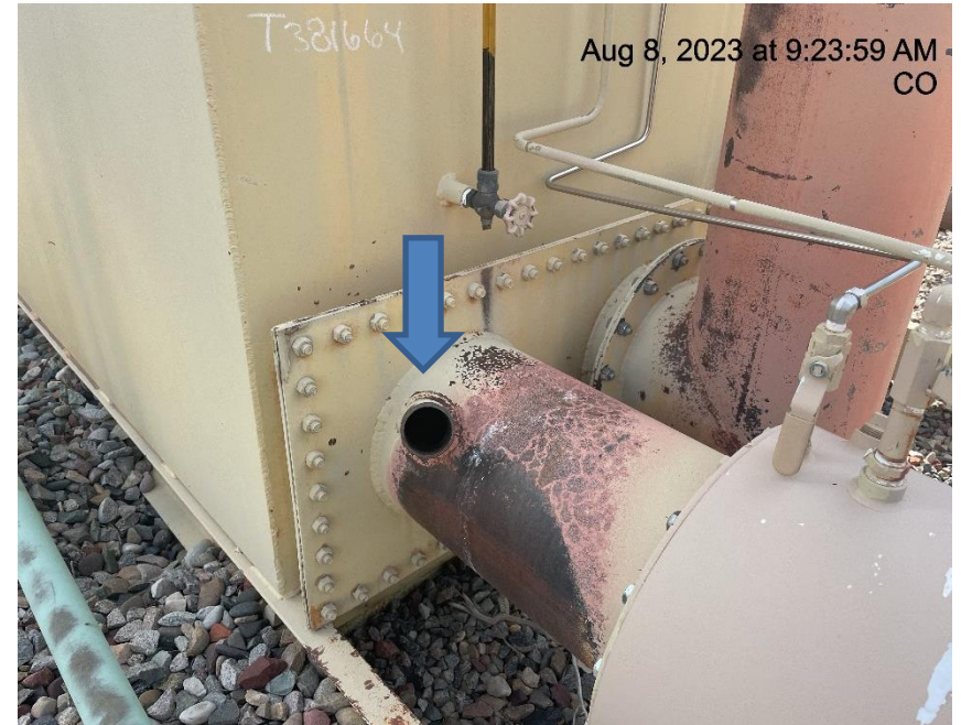
Photo # 5144 Burner missing cap/wildlife hazard
