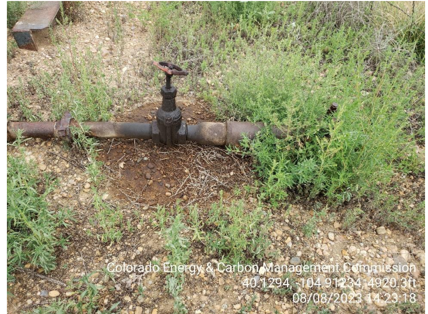
Photo 4 Stained soil at the WH flow line valve, Undesirable vegetation.
