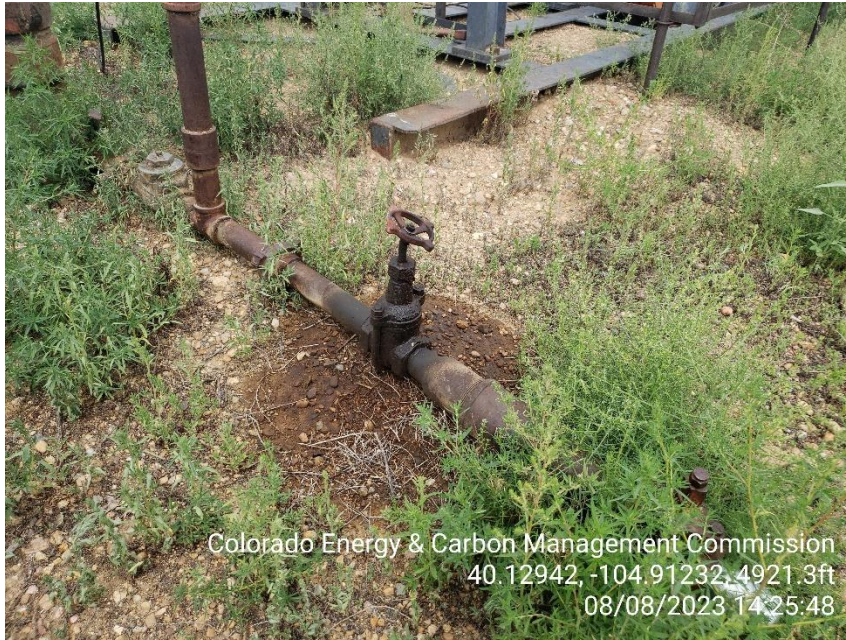
Photo 5 Stained soil at the WH flow line valve, Undesirable vegetation .
