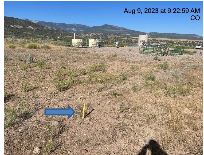
Photo # 5444 Improperly marked deadman
