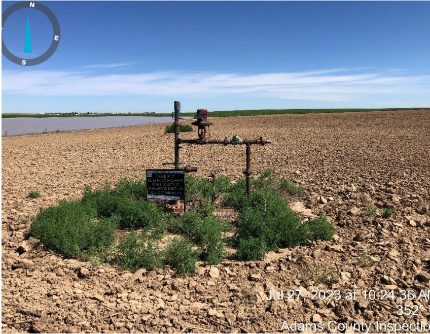
Photo #1 Well head.
