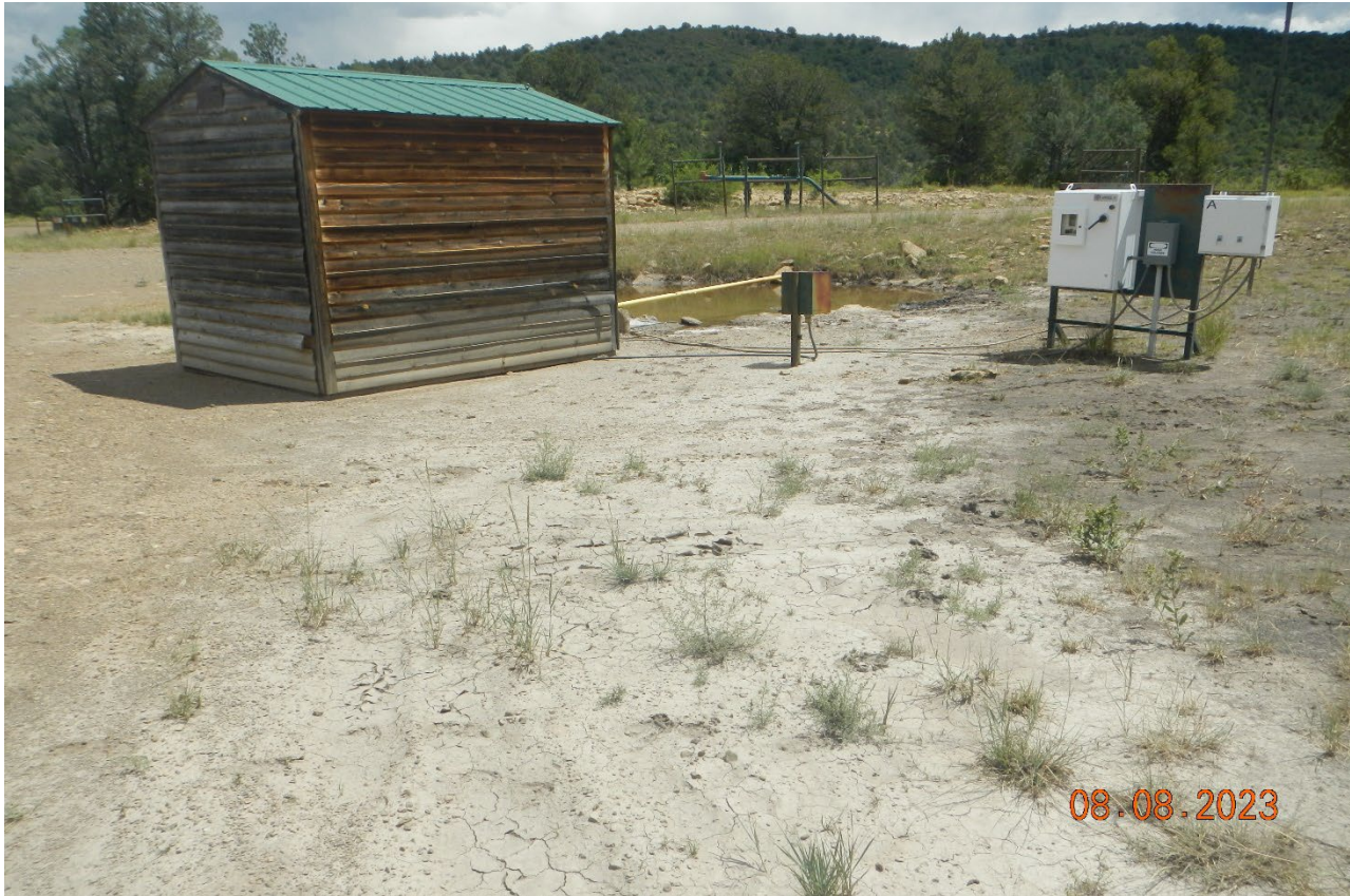
Photo 4. Facing southeast toward the wellsite. There appears to be whitened soils where water may have over flowed toward the red arrow direction.
