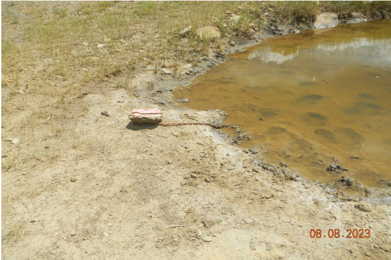
Photo 3. The water level is above freeboard and lays flat n the ground which does not show proper freeboard.
