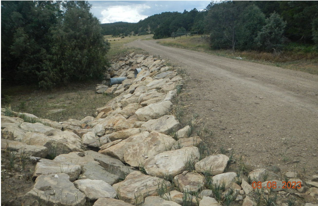
Photo 1. Facing southwest along the access road. The erosion along the drainage and road was repaired and stabilized with rock rip-rap.
