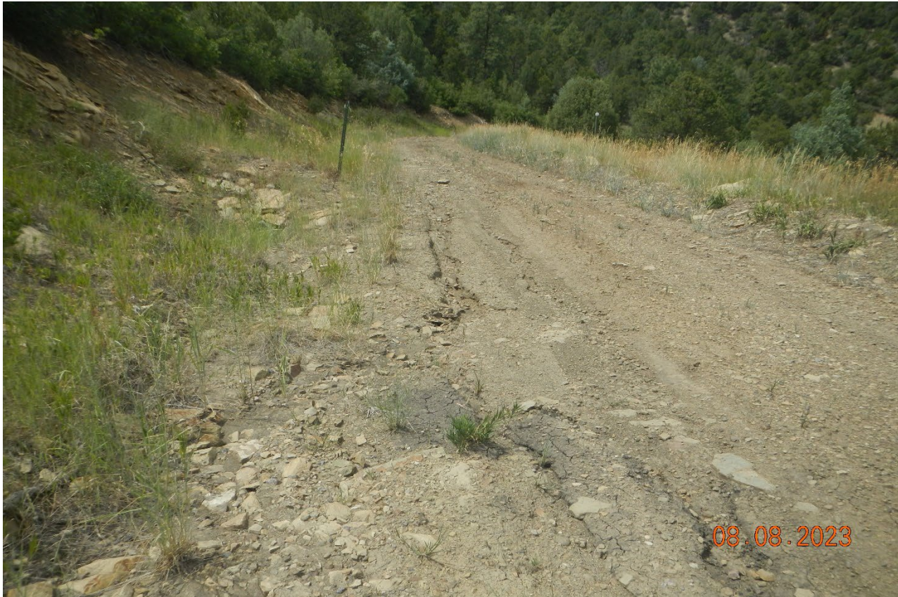
Photo 1. Facing northwest east along the access road traveling from the SECO CANYON 11-22 location. Stormwater is bypassing the culvert causing erosion. The road is not stabilized and gravel has washed away.
