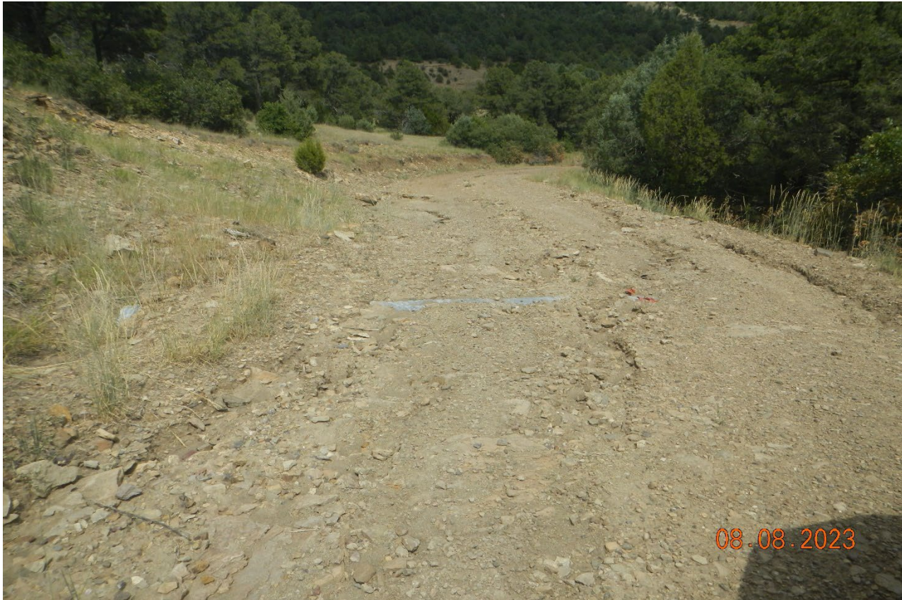
Photo 6. This culvert near the location is partially full of sediment and stormwater is bypassing the culvert causing erosion of the road.
