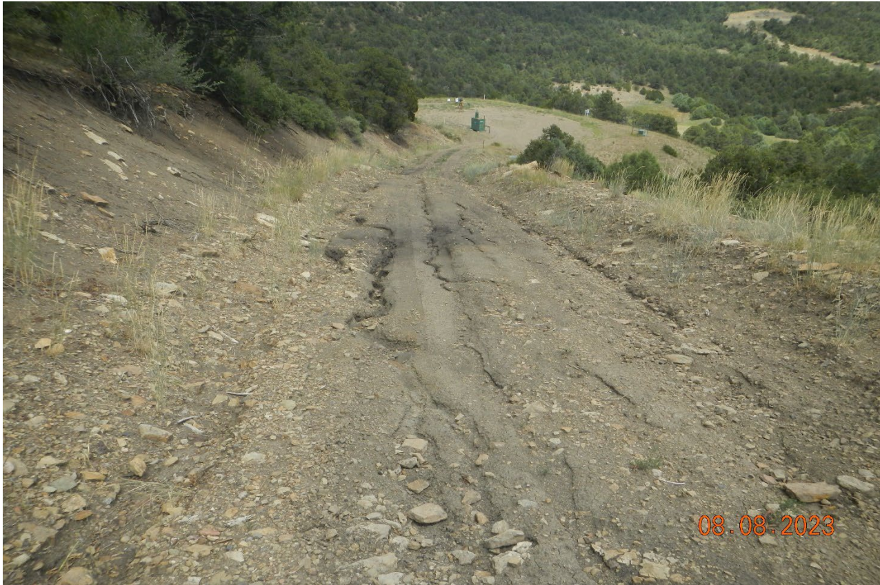
Photo 3. Facing northeast east along the access road toward the location. The road is not stabilized and gravel has washed away.
