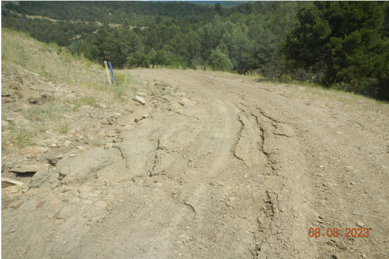
Photo 5. Facing northeast east along the access road near the location. The road is not stabilized and gravel has washed away.
