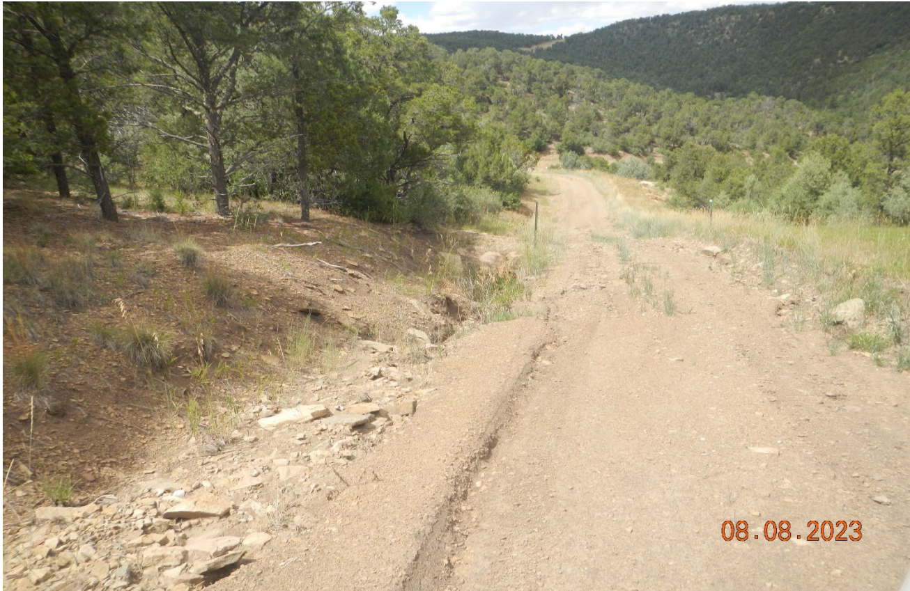
Photo 2. Facing northwest east along the access road traveling from the SECO CANYON 11-22 location. Stormwater is bypassing the culvert causing erosion. There is an erosion gully forming at this culvert.
