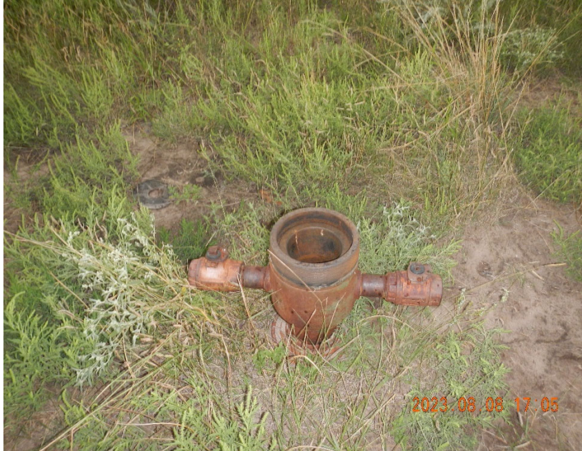
1. View of well open to atmosphere.
