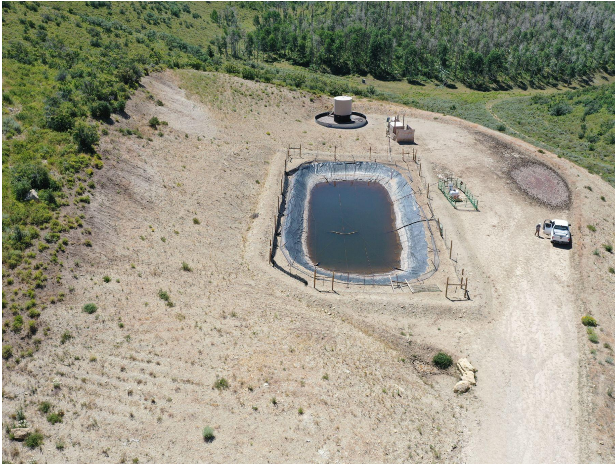
Photo 6: Photo taken with a sUAS. Photo shows pit on the Location; fence remains in disrepair and netting has not been replaced.
