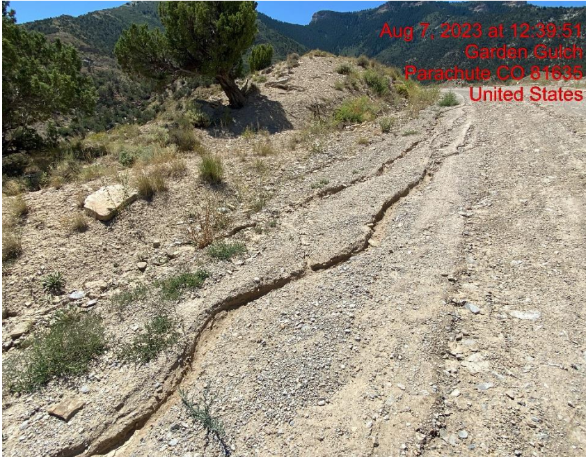
Rill Erosion Cutting Through Lease Road – Photo #05610
