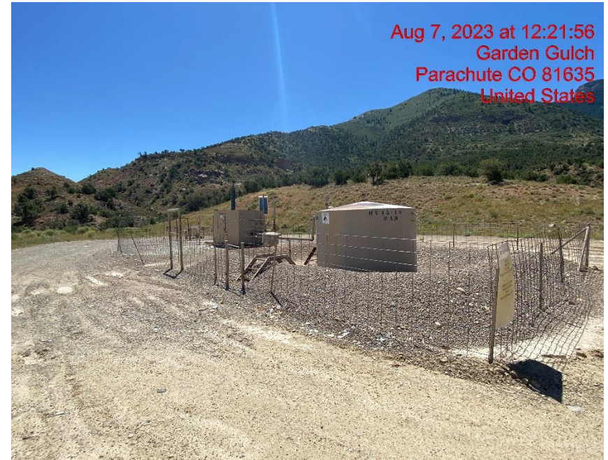
NE Corner of Location – Photo #0
