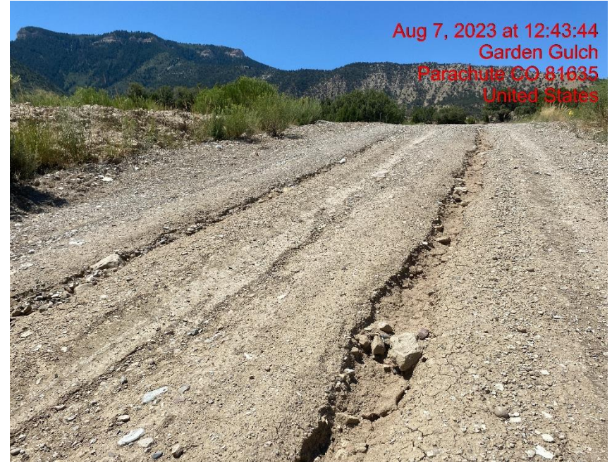
Rill Erosion Cutting Through Lease Road – Photo #05613
