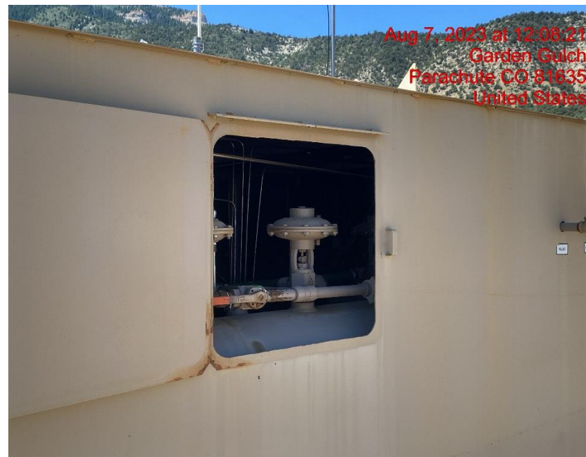
Separator Hatch Unsecured – Photo #05584
