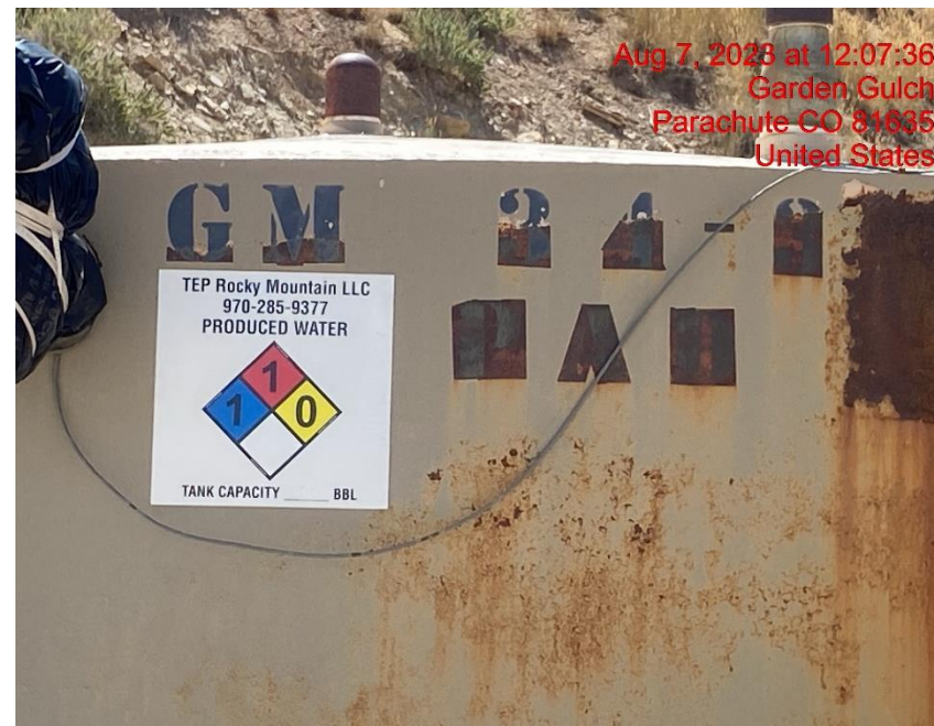
Tank Label Does Not State Capacity – Photo #05581
