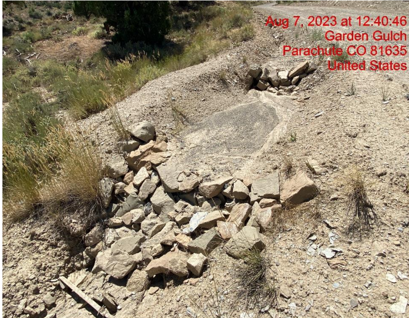
Check Dam Needs Maintenance – Photo #05611
