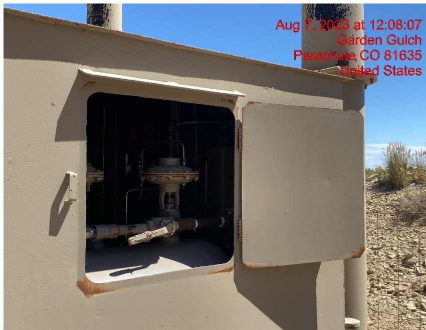
Separator Hatch Unsecured – Photo #05583
