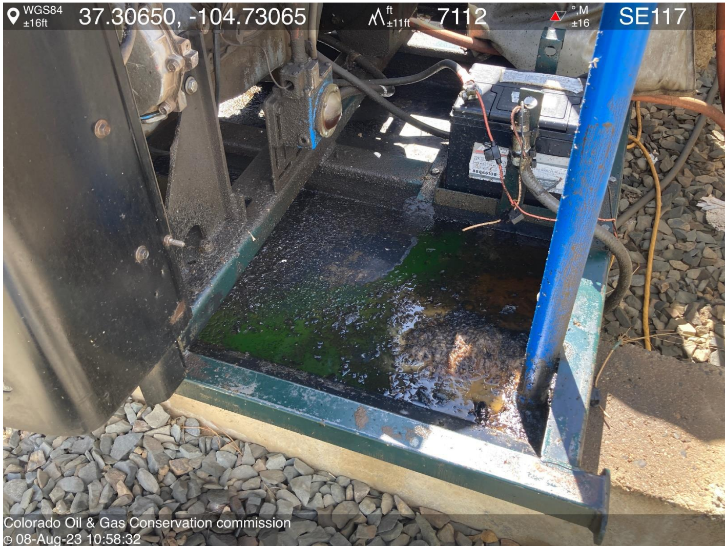
PHOTO 5: ANTIFREEZE AND OILY WASTE IN PRIME MOVER SKID. COMPLY WITH RULE 1002.f.(2)B, Comply with general provisions of the oil and gas act for wildlife protection AND SB-181. CA DATE 8-10-2023.
