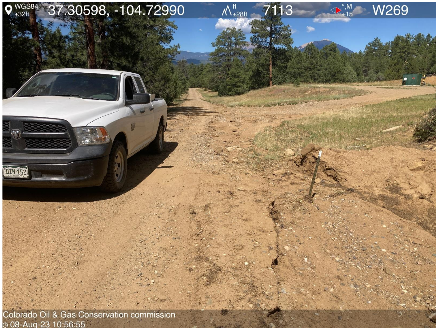
PHOTO 6: CULVERT JUST EAST OF LOCATION ENTRANCE IS FILLED WITH SEDIMENT. Install or repair required BMPs per Rule 1002.f.(2)C. CA DATE 9-9-2023.
