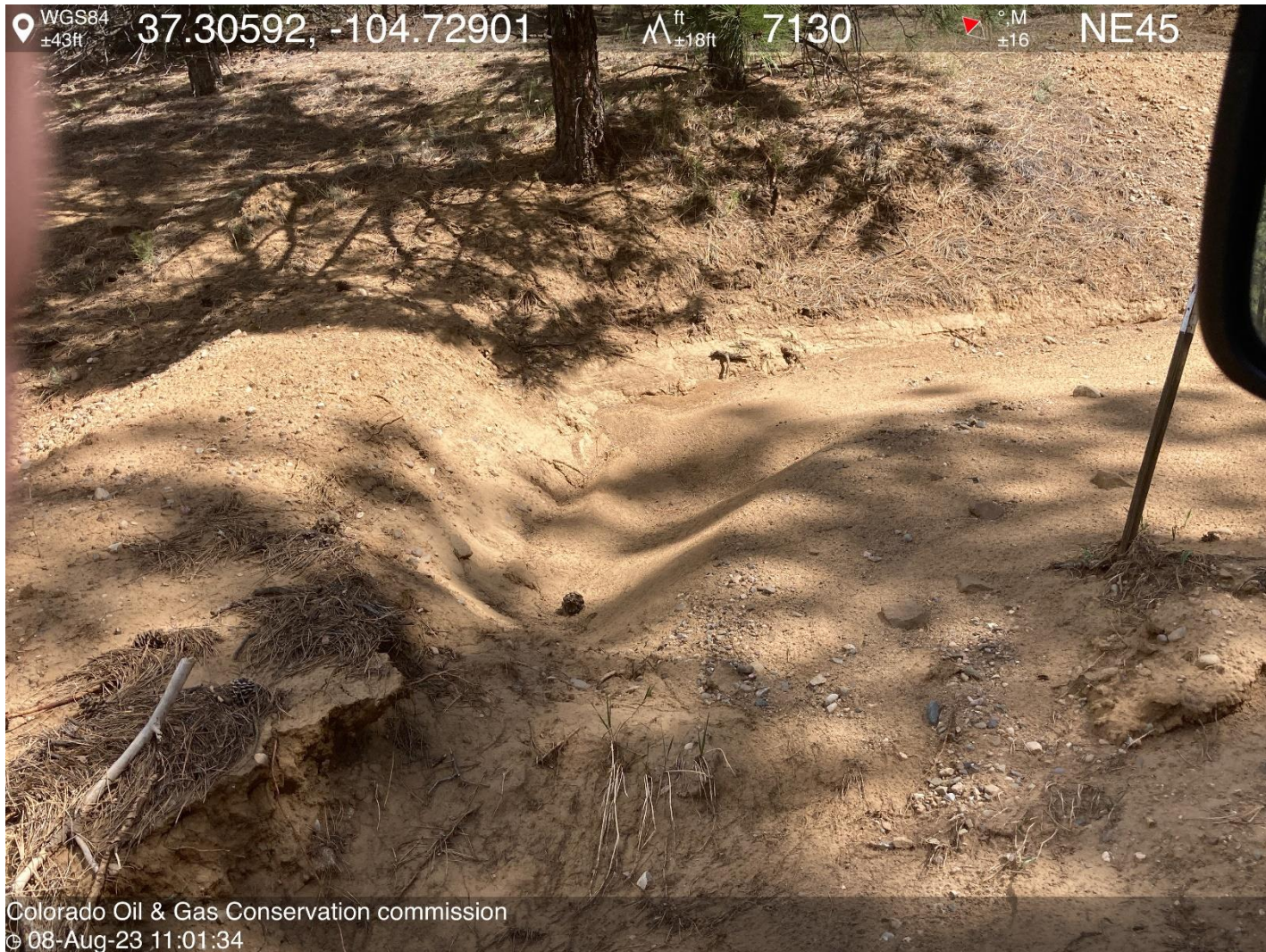
PHOTO 7: CULVERT ABOUT 100 YARDS EAST OF LOCATION ENTRANCE IS FILLED WITH SEDIMENT. Install or repair required BMPs per Rule 1002.f.(2)C. CA DATE 9-9-2023.
