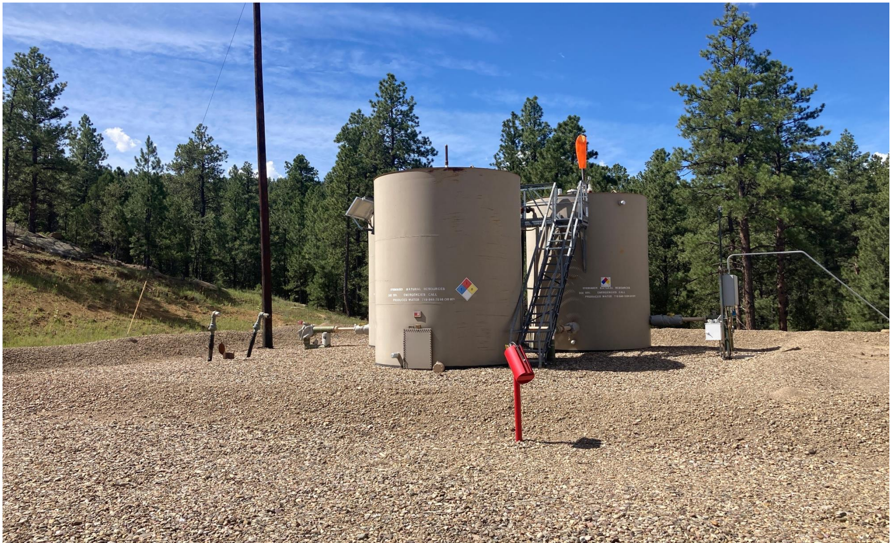
PHOTO 3: TANK BATTERY
