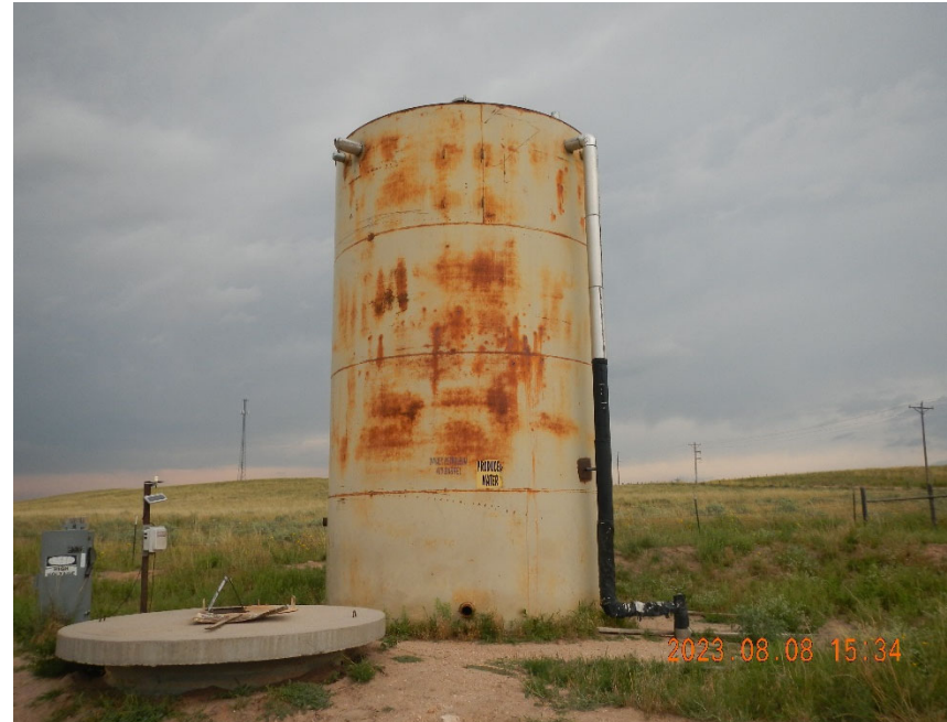
8. View of Steel Tank and Concrete Vault. Note Vegetation.
