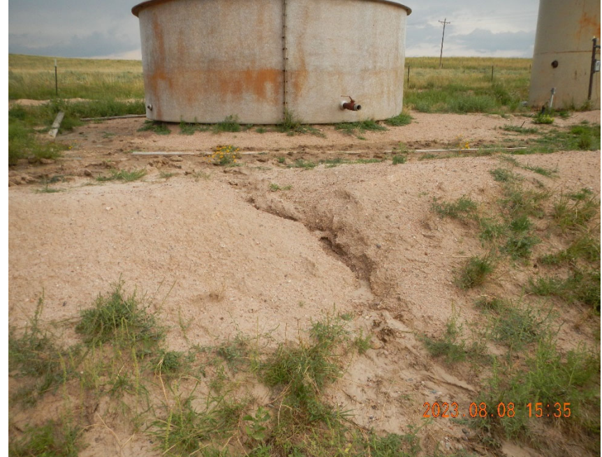
10. Washed out containment berm in SW corner.
