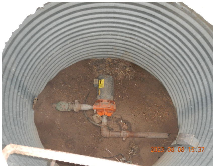
11. Electric pump in bottom of vault.
