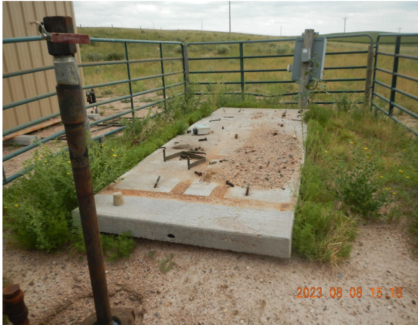
3. Concrete pad and production related debris left at location. Note vegetation.
