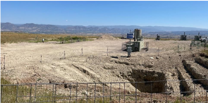
South West corner of location.
