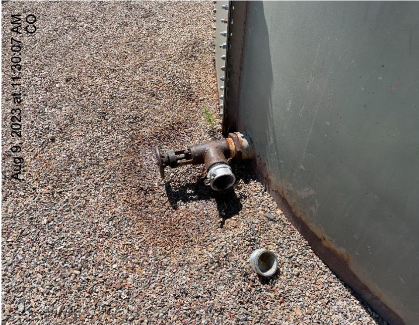
Photo # 5607 Open ended load line & tank valve leaking fluid
