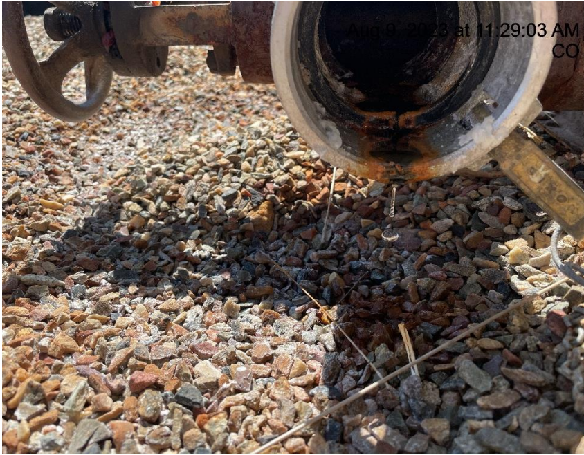
Photo # 5571 Tank valve leaking fluid
