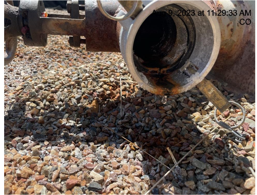
Photo # 5590 Tank valve leaking fluid
