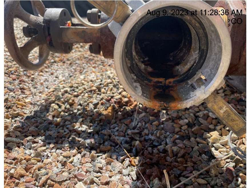
Photo # 5552 Tank valve leaking fluid
