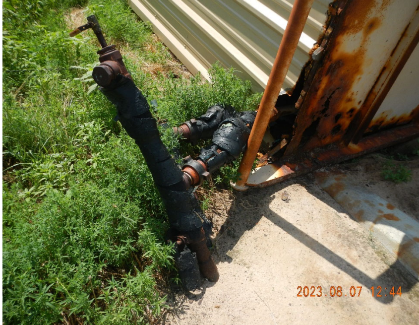
7. View of Meter Run Outlet lines (Gas and water lines).
