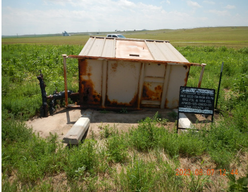
5. View of Meter Shed blown off supports and on its back. Note vegetation.
