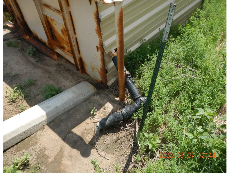
6. View of Meter Run Inlet flowline from the well.
