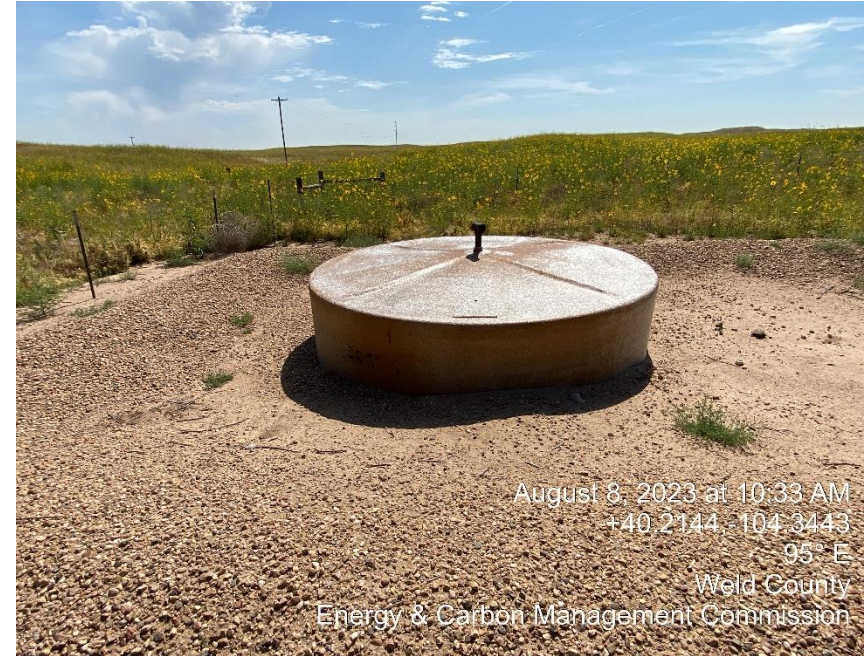
Pit missing capacity and NFPA placards
