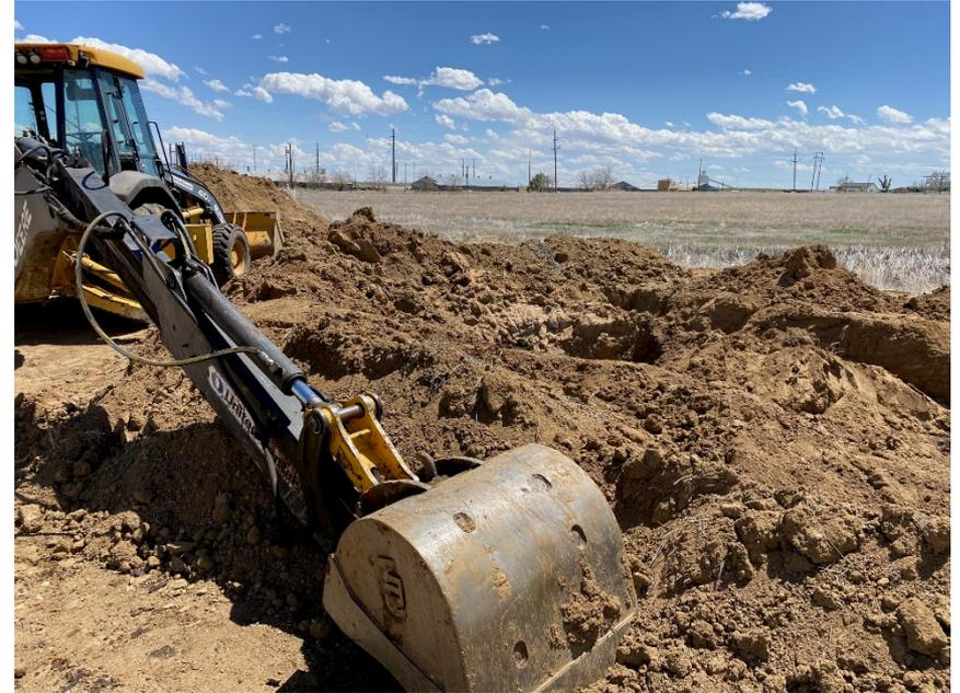
**The Shannon-Roberts-61N68W 26NENE Tank Battery is in the CECMC Orphan Well Program. Stained soils were observed beneath the produced water tank and the production AST at the Tank Battery during decommissioning activities on 05/12/2023.**
