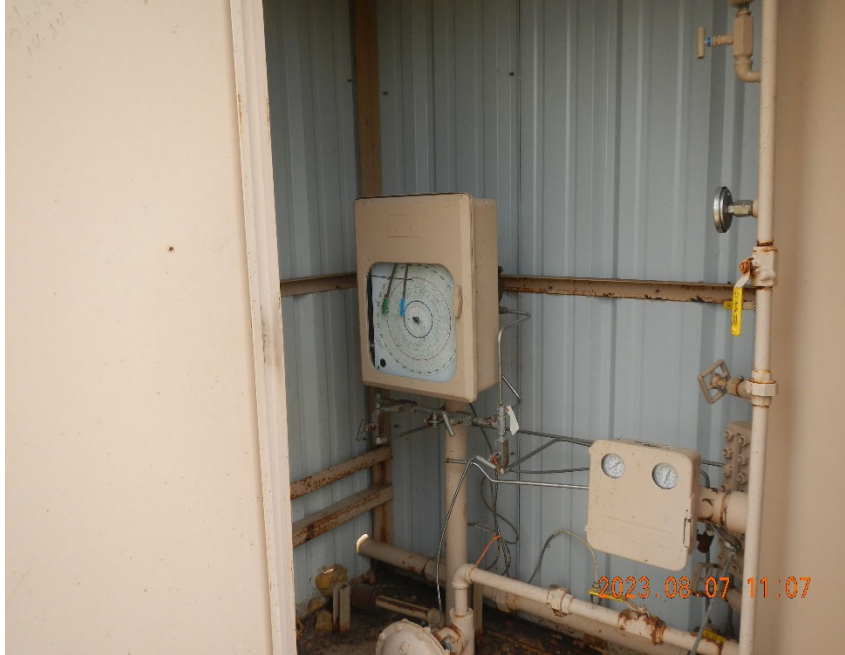
3. Gas Meter Run inside Meter Shed.
