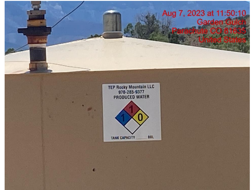
Tank Label Missing Capacity – Photo #05569
