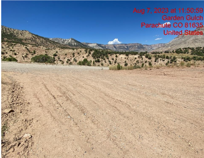
Insufficient Vehicle Tracking BMPs at Location Entrance/Exit – Photo #05571
