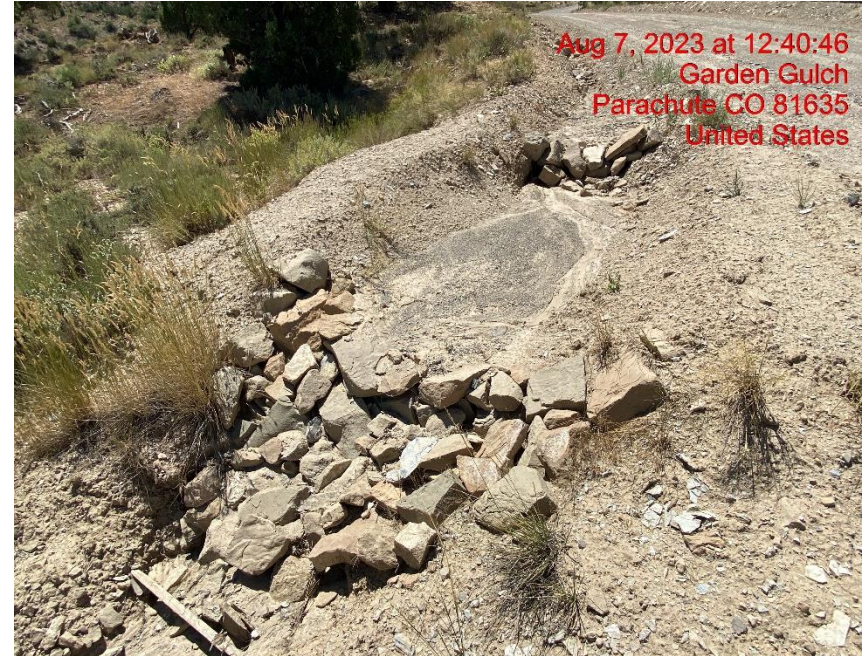
Check Dam Needs Maintenance – Photo #05611
