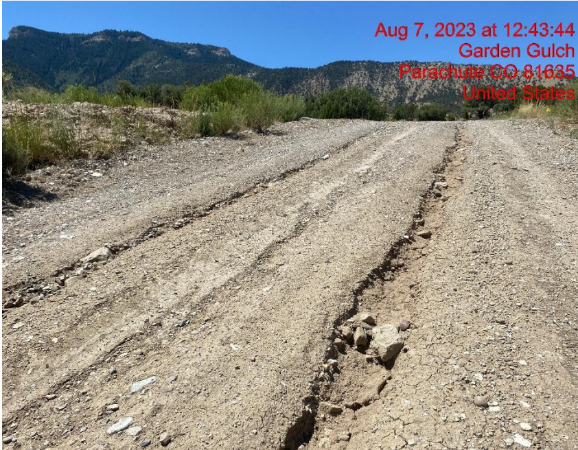
Rill Erosion Cutting Through Lease Road – Photo #05613
