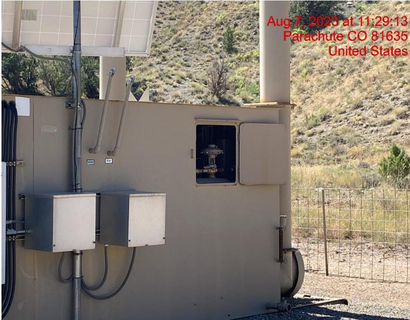
Separator Hatch Unsecured – Photo #05551
