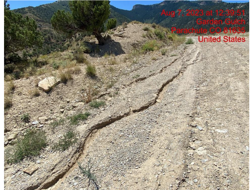
Rill Erosion Cutting Through Lease Road – Photo #05610
