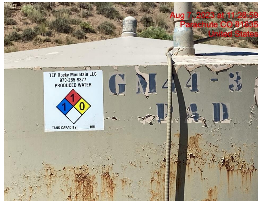
Tank Label Missing Tank Capacity – Photo #05550
