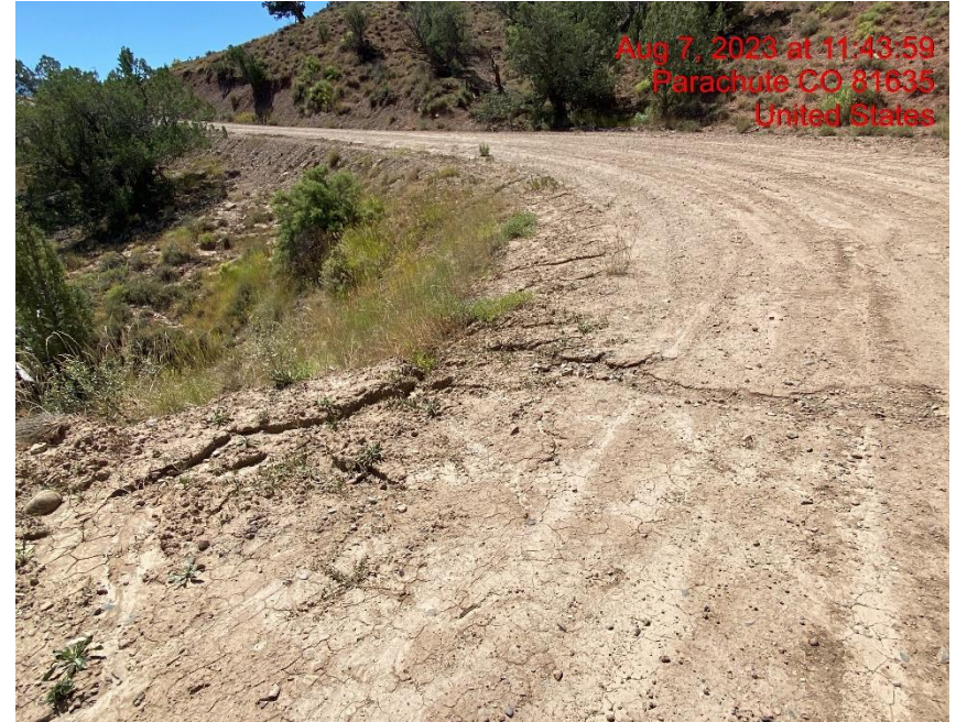
Rill Erosion Transporting Sediment to Nearby Watershed – Photo #05555
